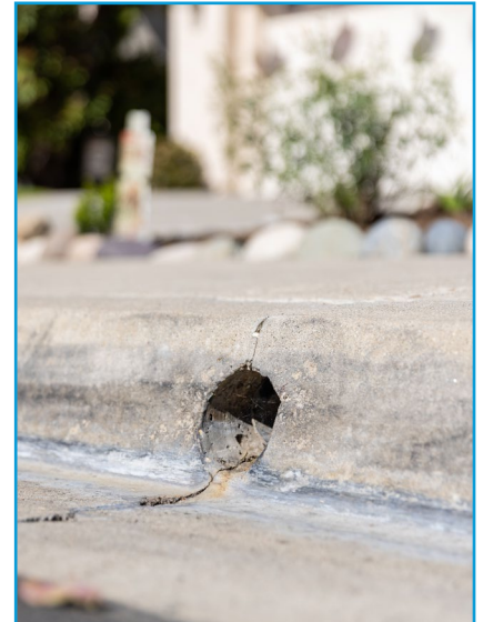
Curb cut with proper drainage.
