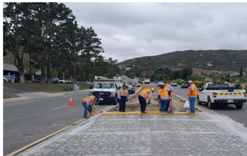
City crews constructing a center median.
