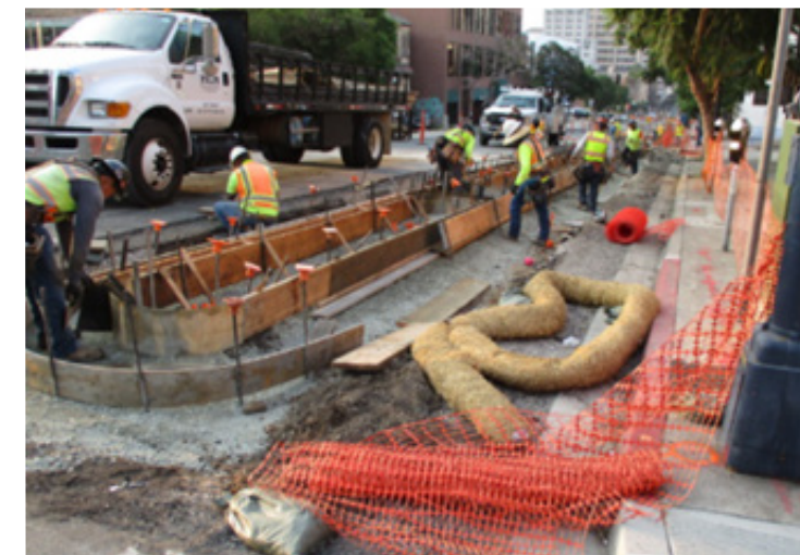
Construction of the 5th Street Bikeway in Downtown San Diego
