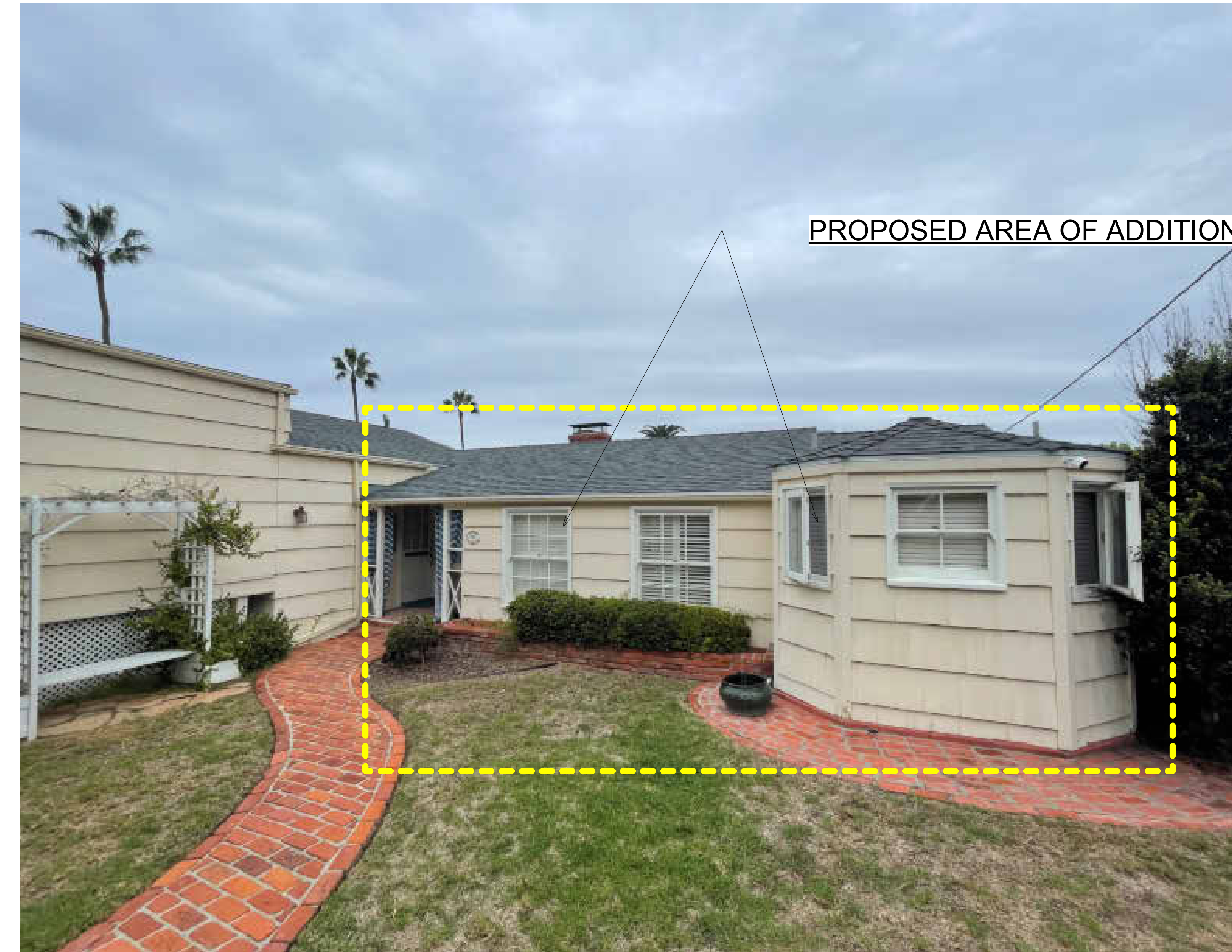
7988 ROSELAND DRIVE SOUTH ELEVATION FROM YARD
