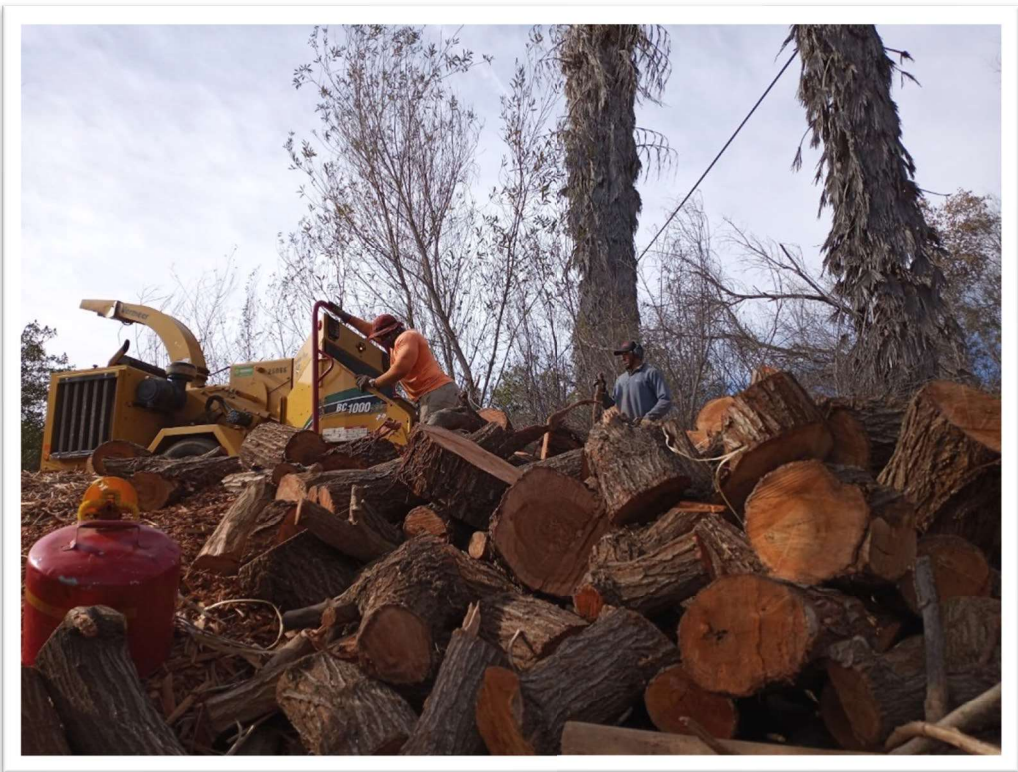
Trees Removed and Chipped
