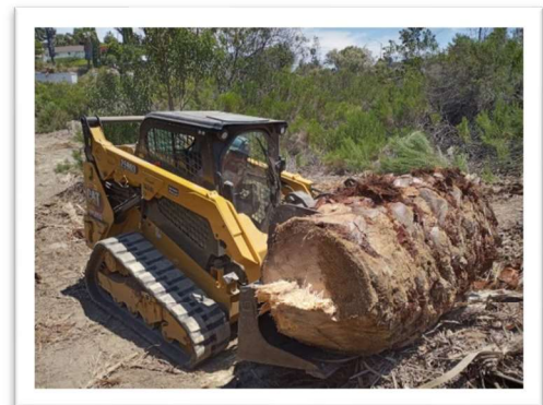
Using Heavy Equipment to Clear Site
