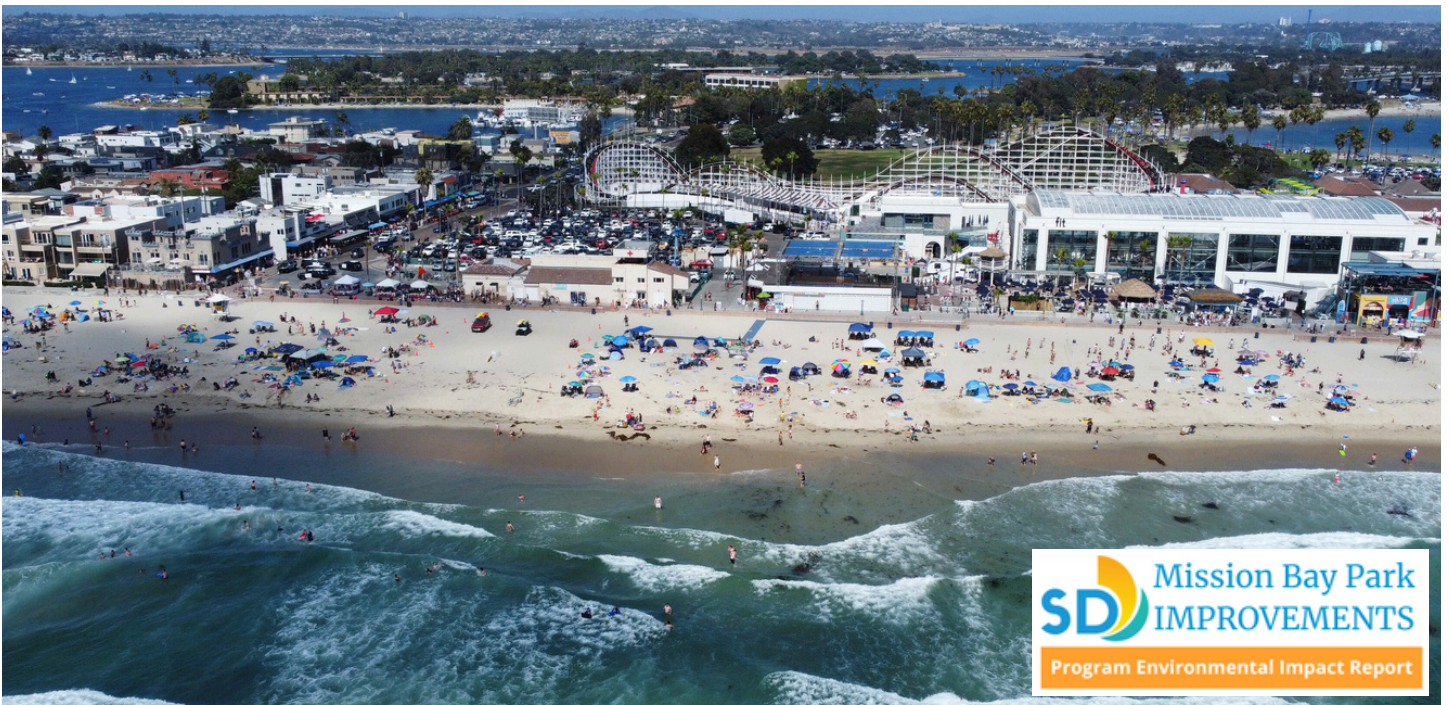
The original segment of the seawall near Belmont Park was upgraded in 2015.
