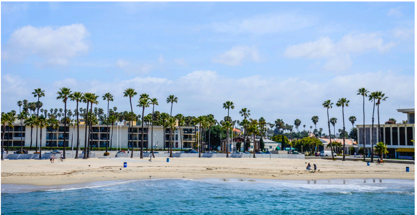
The seawall helps protect Mission Beach from coastal erosion.
