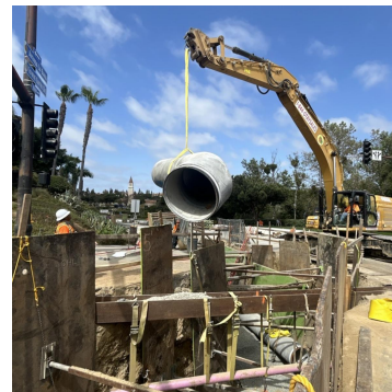
Pipeline installation occurs in the westbound lanes on Nobel Drive.
