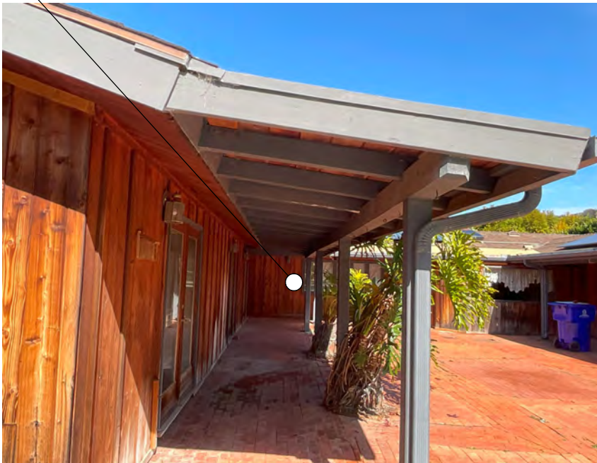
WEST SIDE OF INTERIOR COURT YARD
