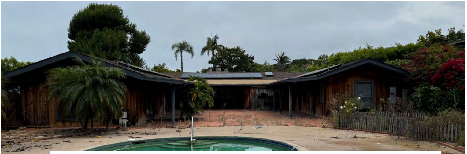
PHOTO OF (E) REAR (SOUTH) FACING VIEW OF RESIDENCE
