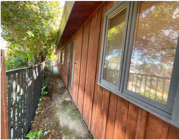
WEST FACING EXTERIOR SIDERYARD WALL LOOKING TOWARD THE STREET
