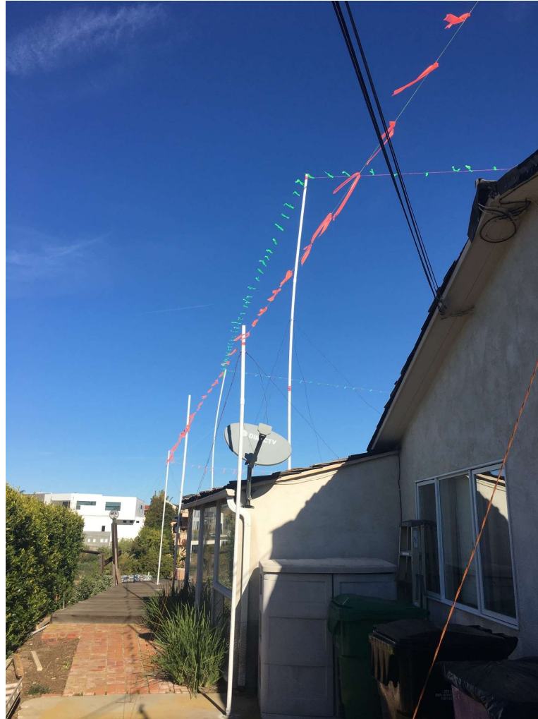
West Lot Line View
