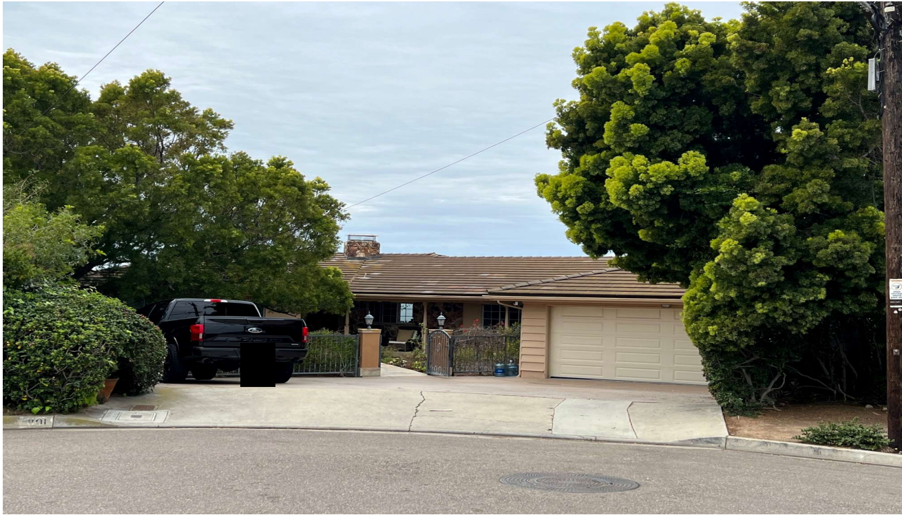
Picture 5 – 2 stories, 1 below street level
