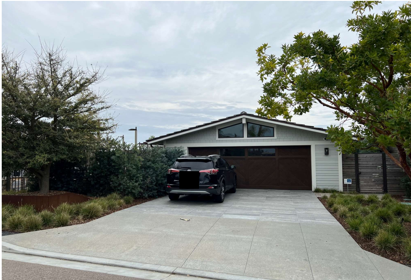
Picture 7 – 2 stories, 1 below street level
