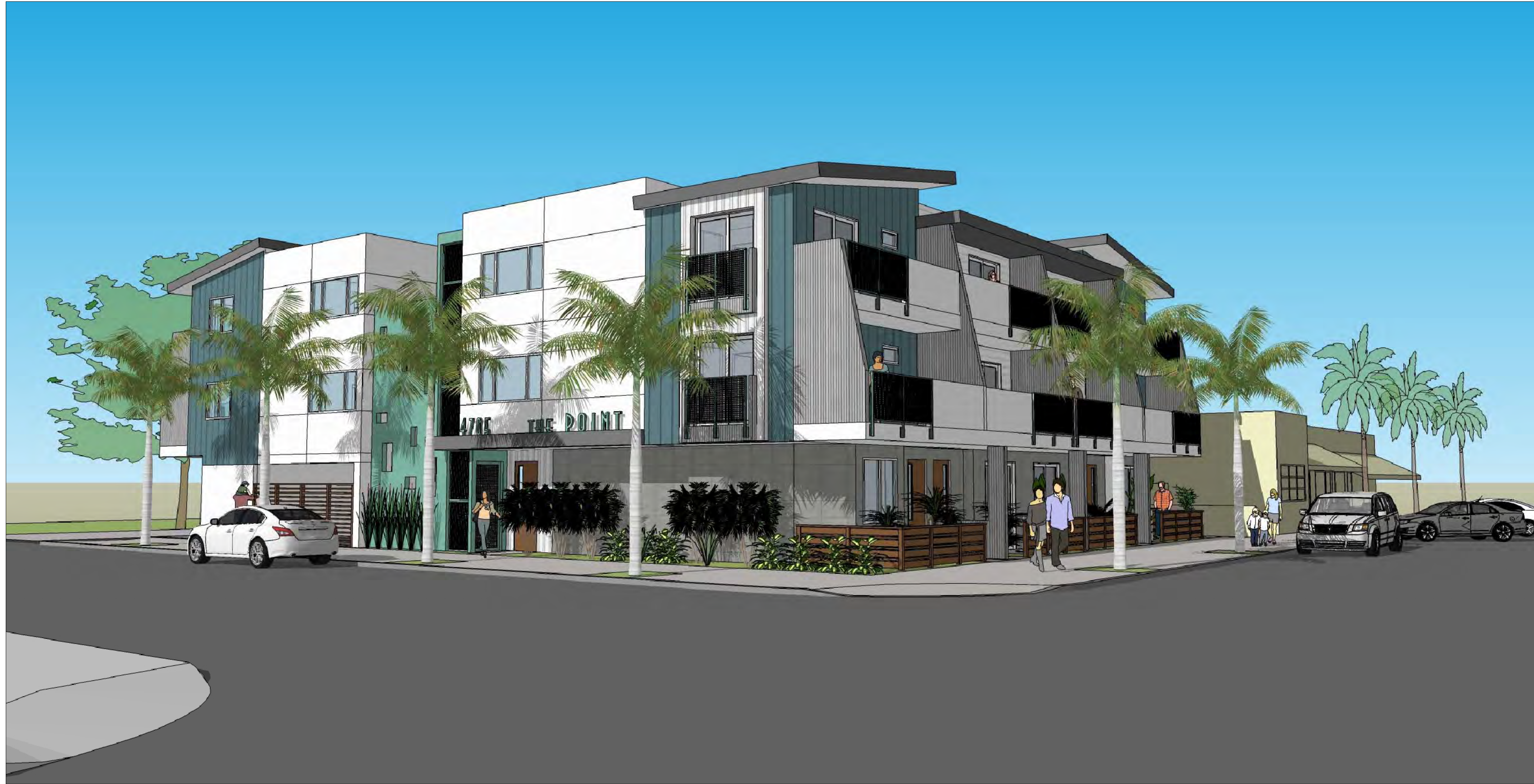
ARTISTIC RENDERING - CONCEPT ONLY. REFER TO CONSTRUCTION PLANS FOR DETAILS, MEANS, AND METHODS.
