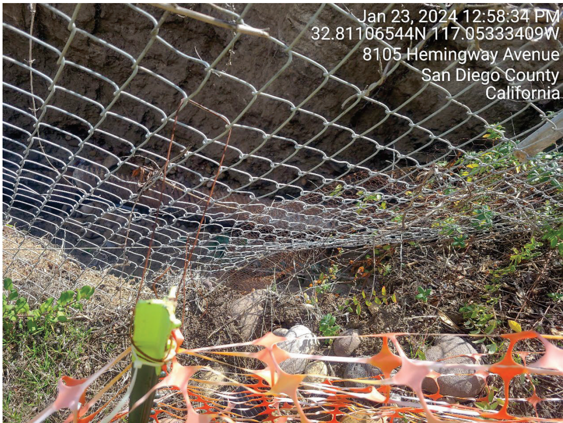
Sinkhole extending into 8105 Hemingway Ave
