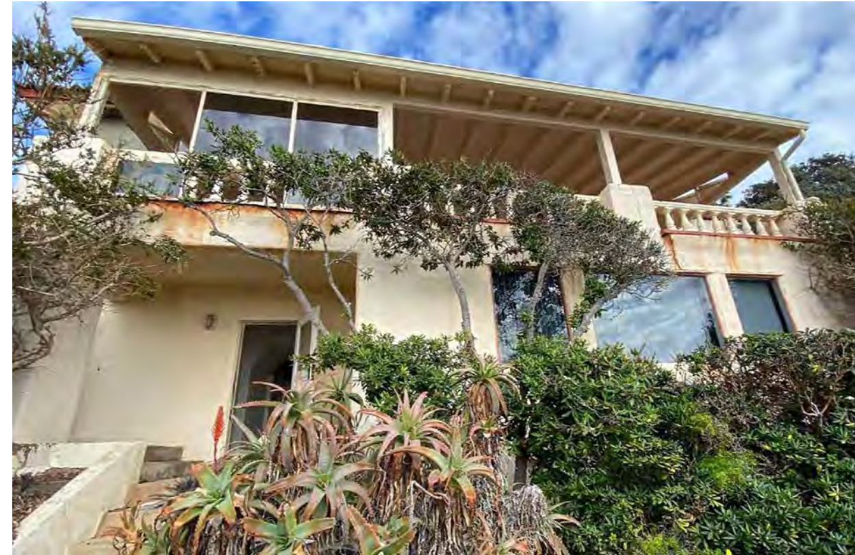
Rear of existing single-dwelling unit
