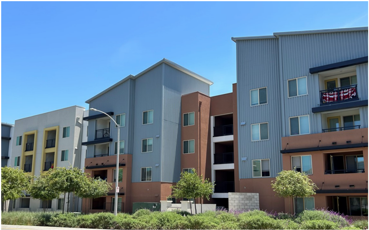
Residential development in Mira Mesa.
