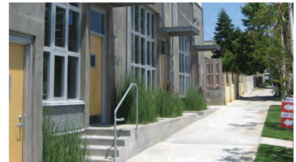
Provide space for an entry and front landing between the public sidewalk and the private entryway
