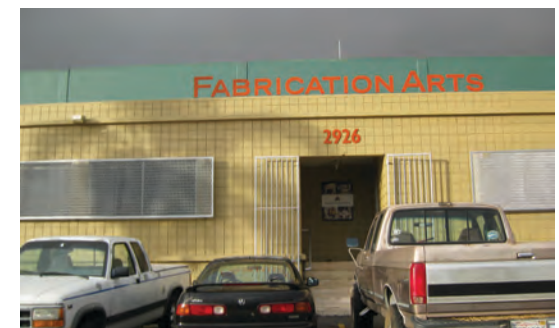
Older industrial buildings in predominantly residential areas can be adaptively reused for commercial purposes
