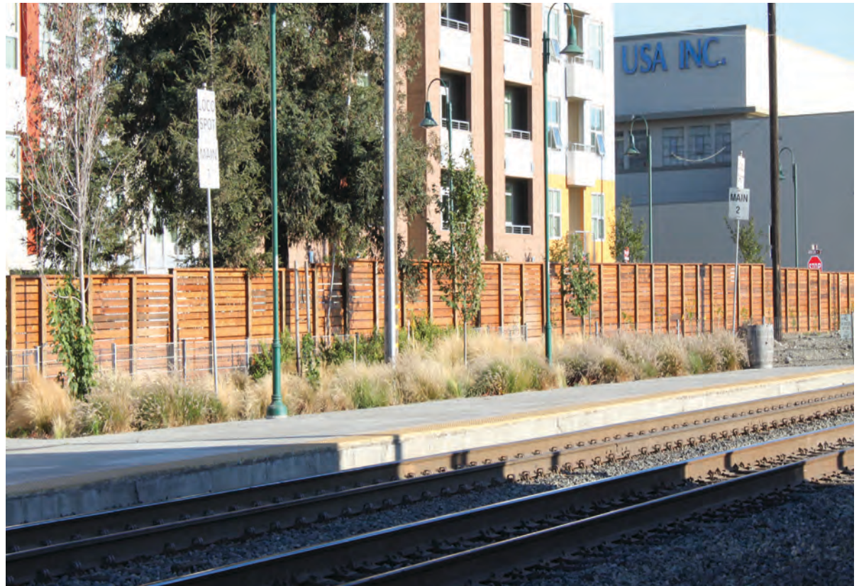
Treat rail facing facades as primary facades
