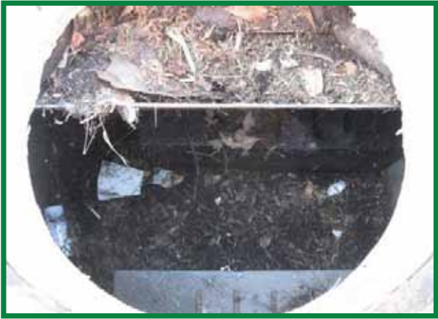
Assess Pollutant Loading in Catch Basin Filter and Sediment Chamber
