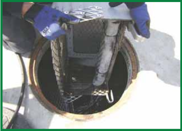
Remove Catch Basin Filter
