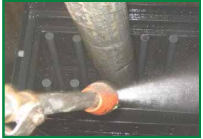
Spray Down and Clean Cartridge Filter Housing
