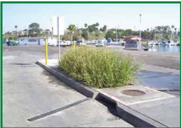
Evaluate Vegetation and Trim if Needed. Maintenance Complete.
