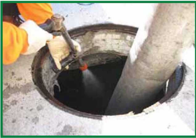
Vacuum out the Sediment Chamber
