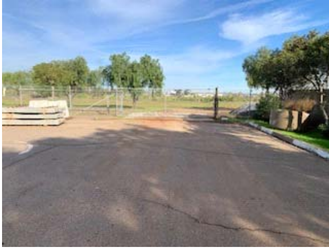
1. View north of the Site access gate from the trolley station parking lot.
