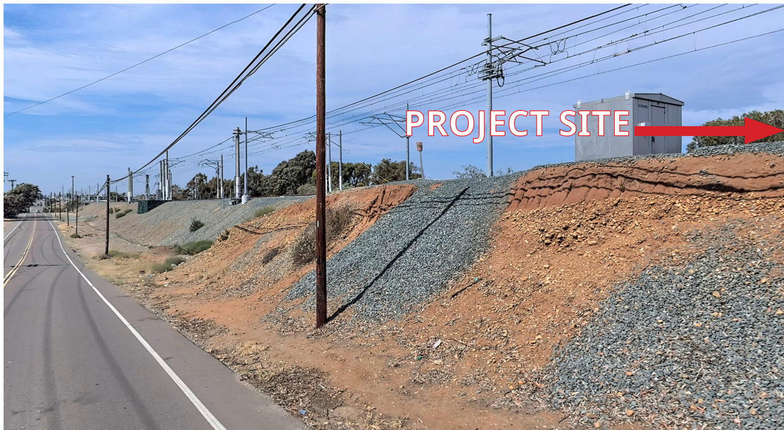
SD&AE/Trolley Track Berm (Project site Lies to the east.)
