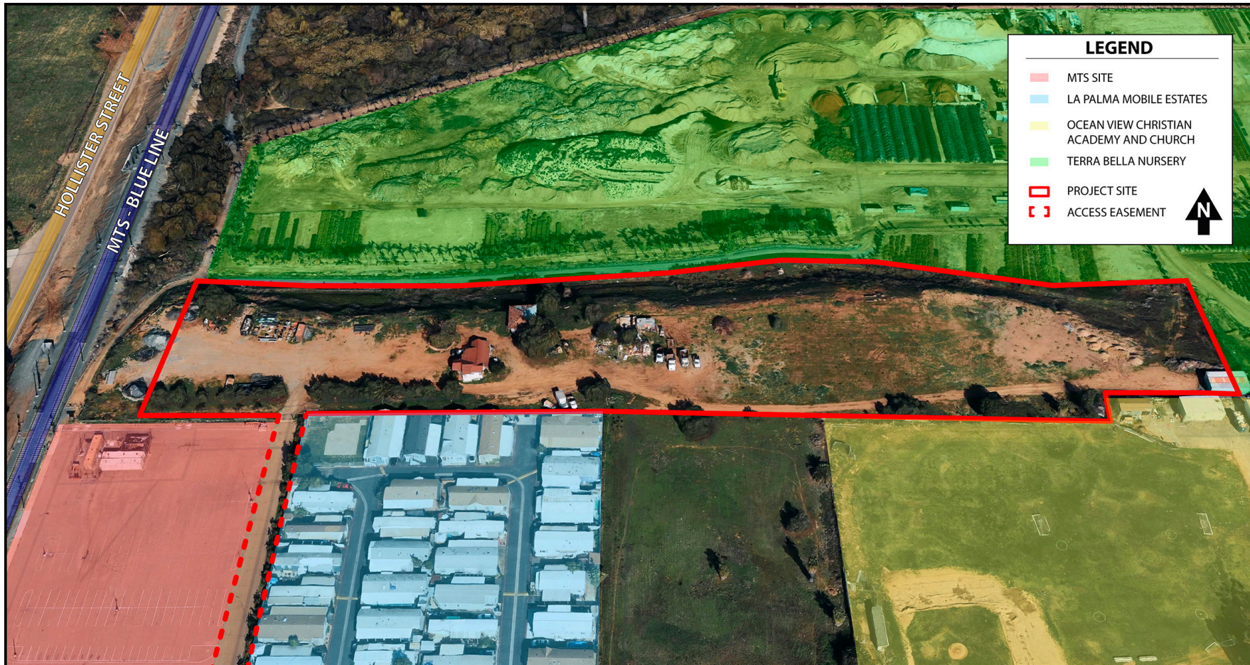
Figure 5.16-1. Existing Site Conditions - Close-up
