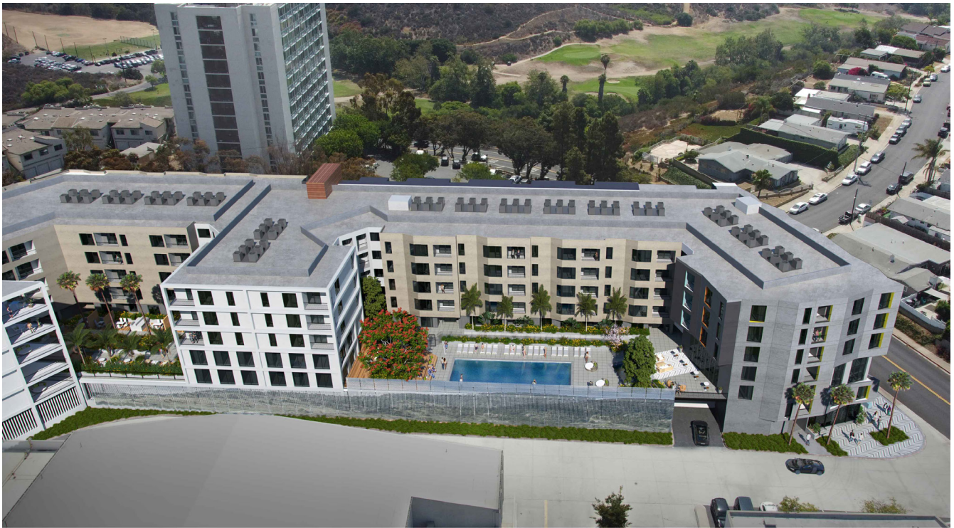
ABOVE SPROUTS LOOKING EAST
