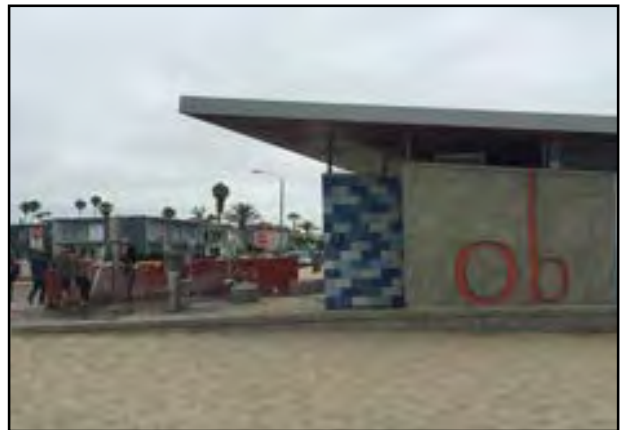
Ocean Beach public restrooms and showers.
