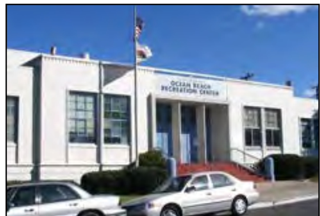
Indoor recreation and community meeting rooms are provided at the existing Ocean Beach Recreation Center.
