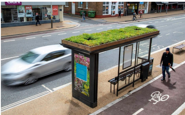
Example of Moss Stop. Green bus stops can make public transit systems more climate ready, helping to reduce urban heat, improve air quality, and absorb rainwater.
