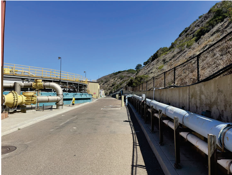
Site overview of proposed ground disturbance area behind digesters, facing north.
