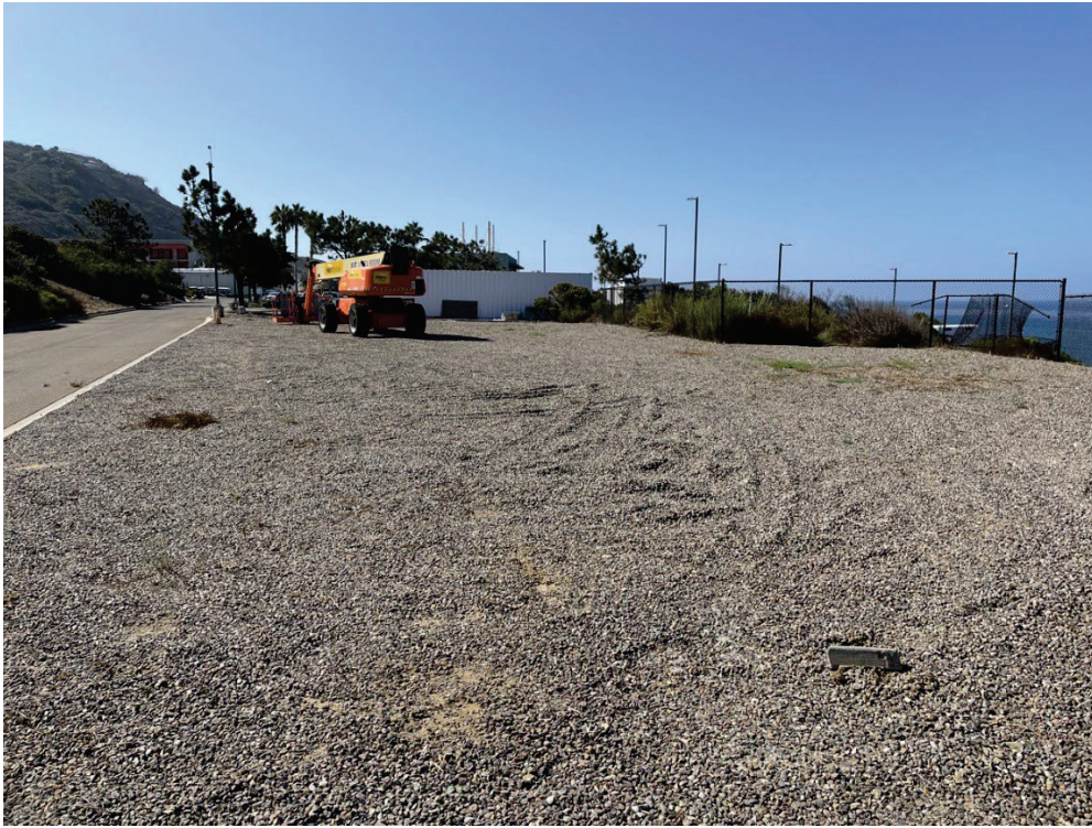
Parking area at south end of facility, facing south.
