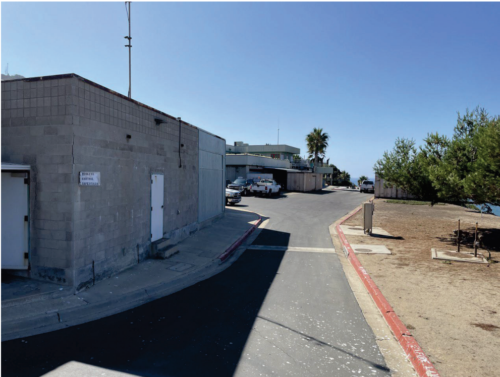
North end of APE with existing drains, facing south.
