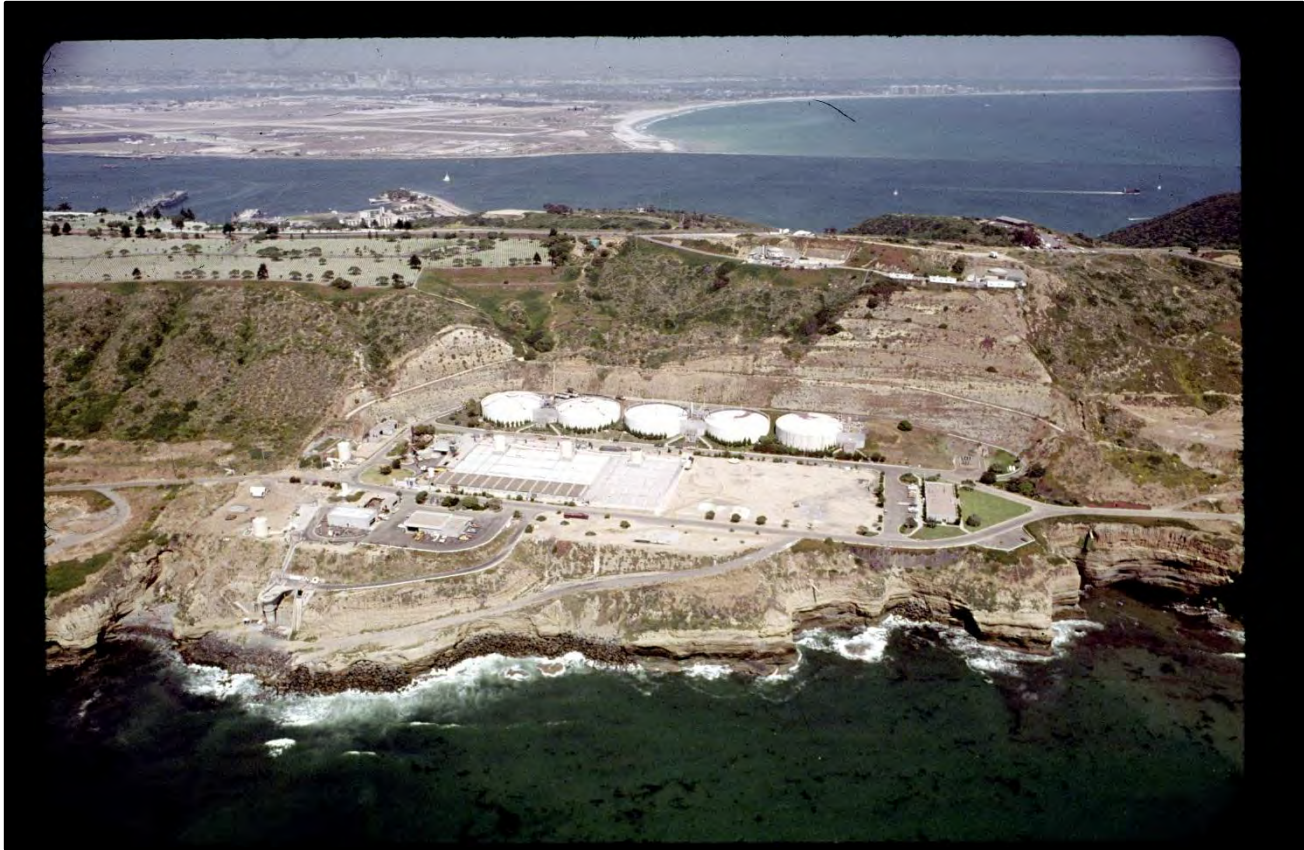
Figure B-3.2. Oblique Aerial, May 1979 (N32 40.75, W117 15.26)
