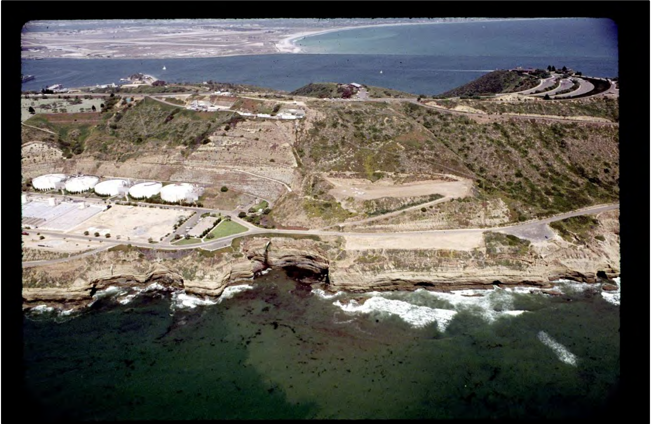
Figure B-3.1. Oblique Aerial, May 1979 (N32 40.60, W117 15.21)
