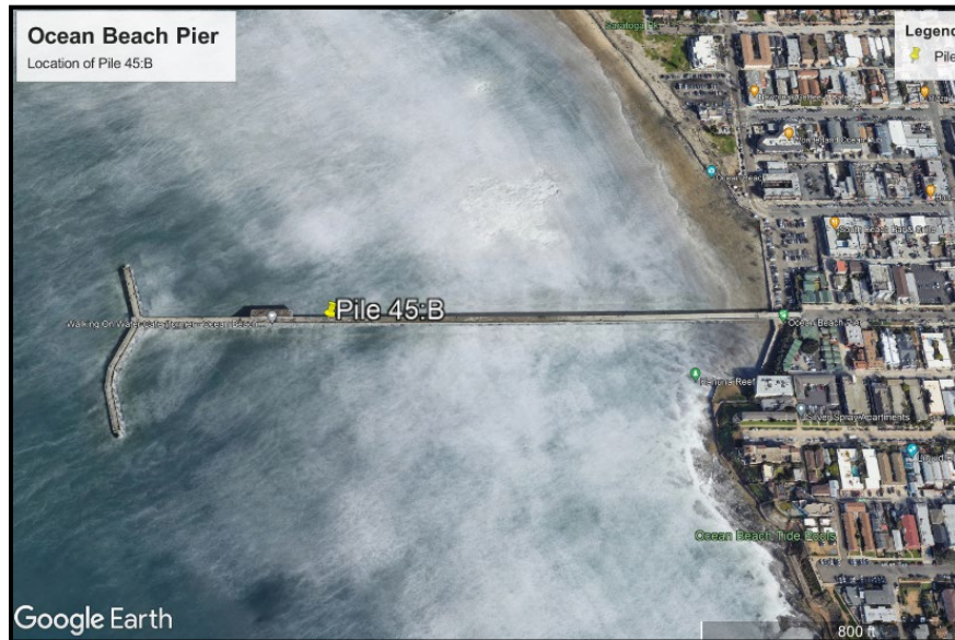
Figure 4: OB Pier Aerial Image showing the missing Pile 45:B.
