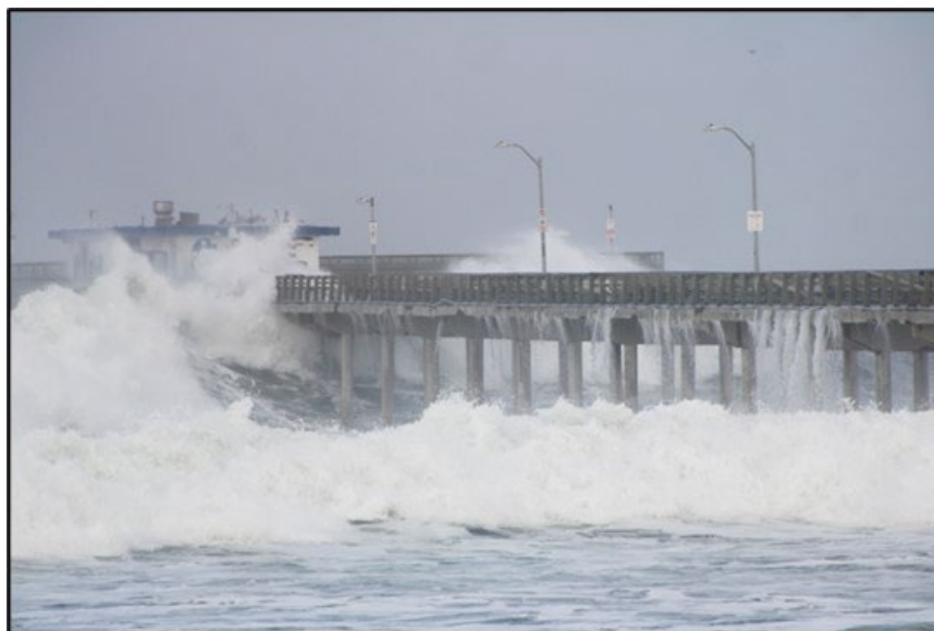
Photo 2: December 28th-29th, 2023, storm event impacting the OB Pier. Note that the broken wave overtops the pier and completely engages the underside of the deck and pile cap.
