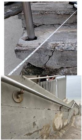
East Stairs Failure of cement steps at sand; large and unsafe 2-3 ft drop-off and access to beach.
