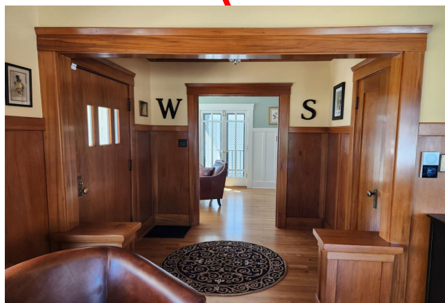
Entry gumwood wainscoting, and door and window surrounds
