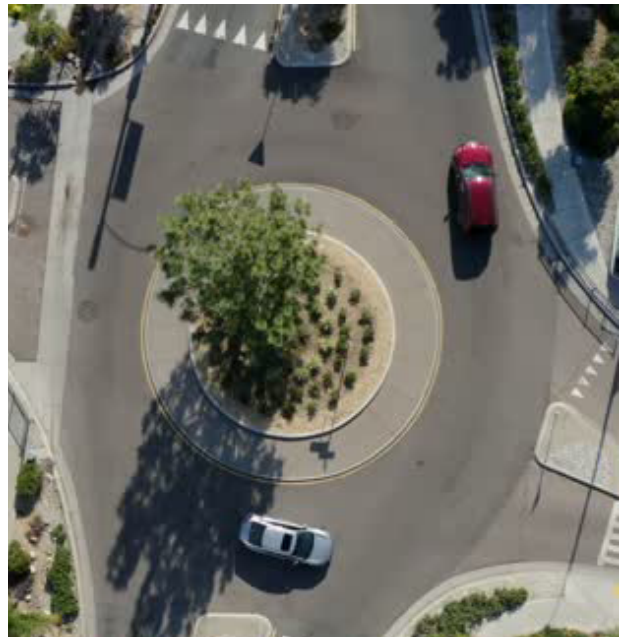
Roundabouts, such as this traffic calming measure in the Bird Rock community, reduce vehicle speeds.
