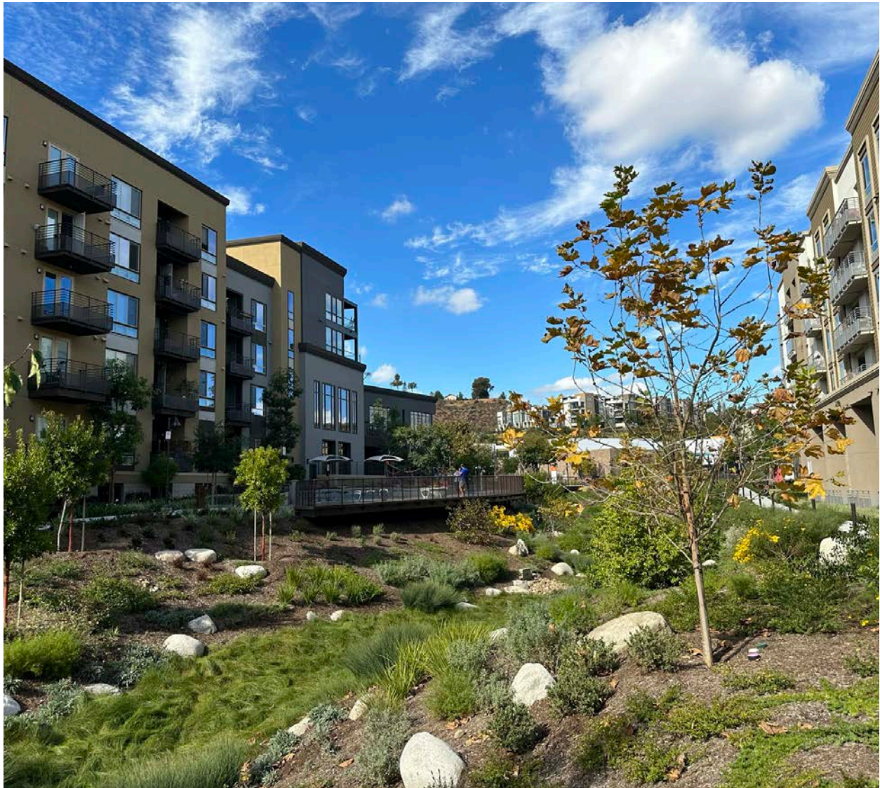
A rain garden integrated into new development in Mission Valley.
