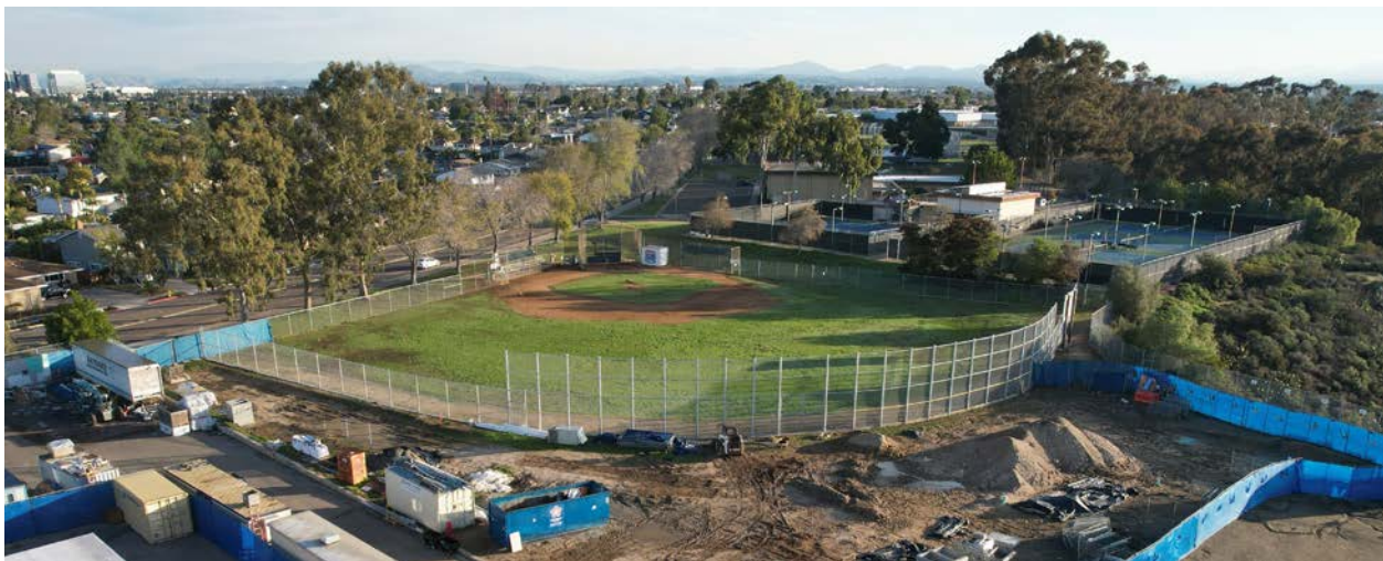
Improvements underway at Spreckels Elementary School in the University Community.
