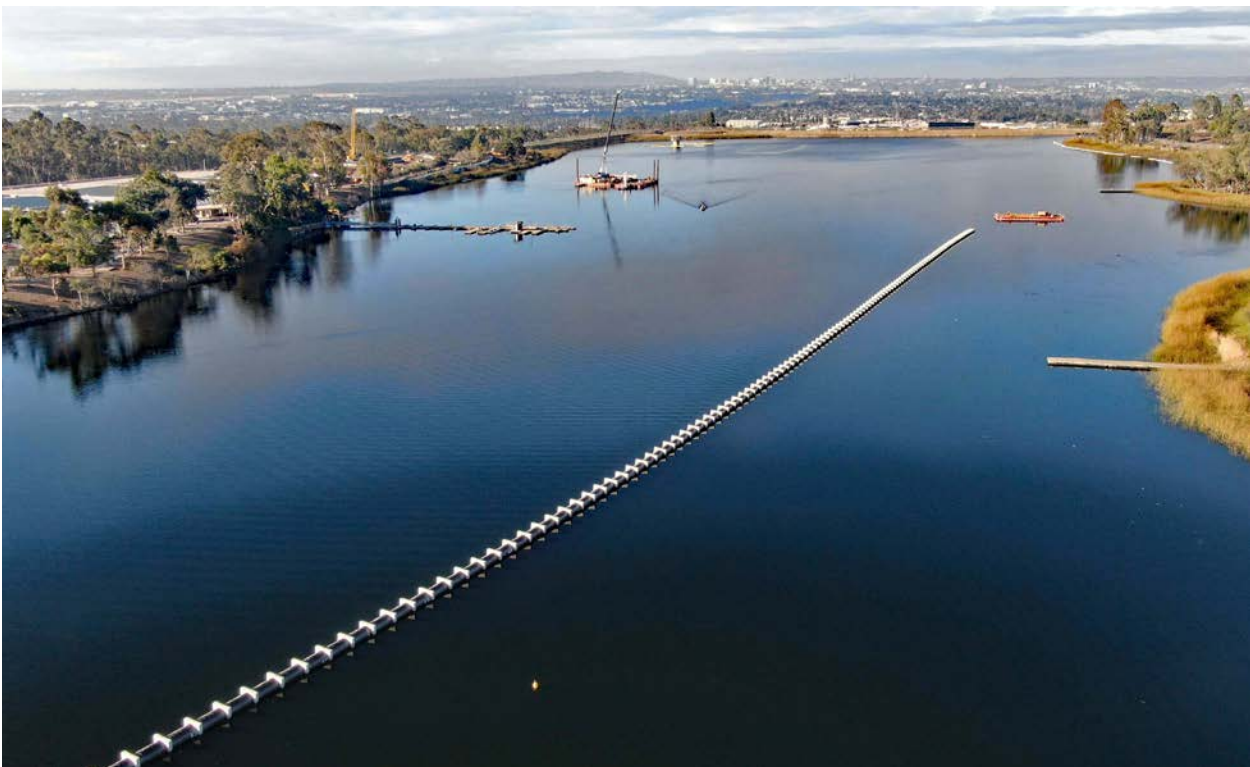
Pure Water project subaqueous pipeline (top and bottom).
