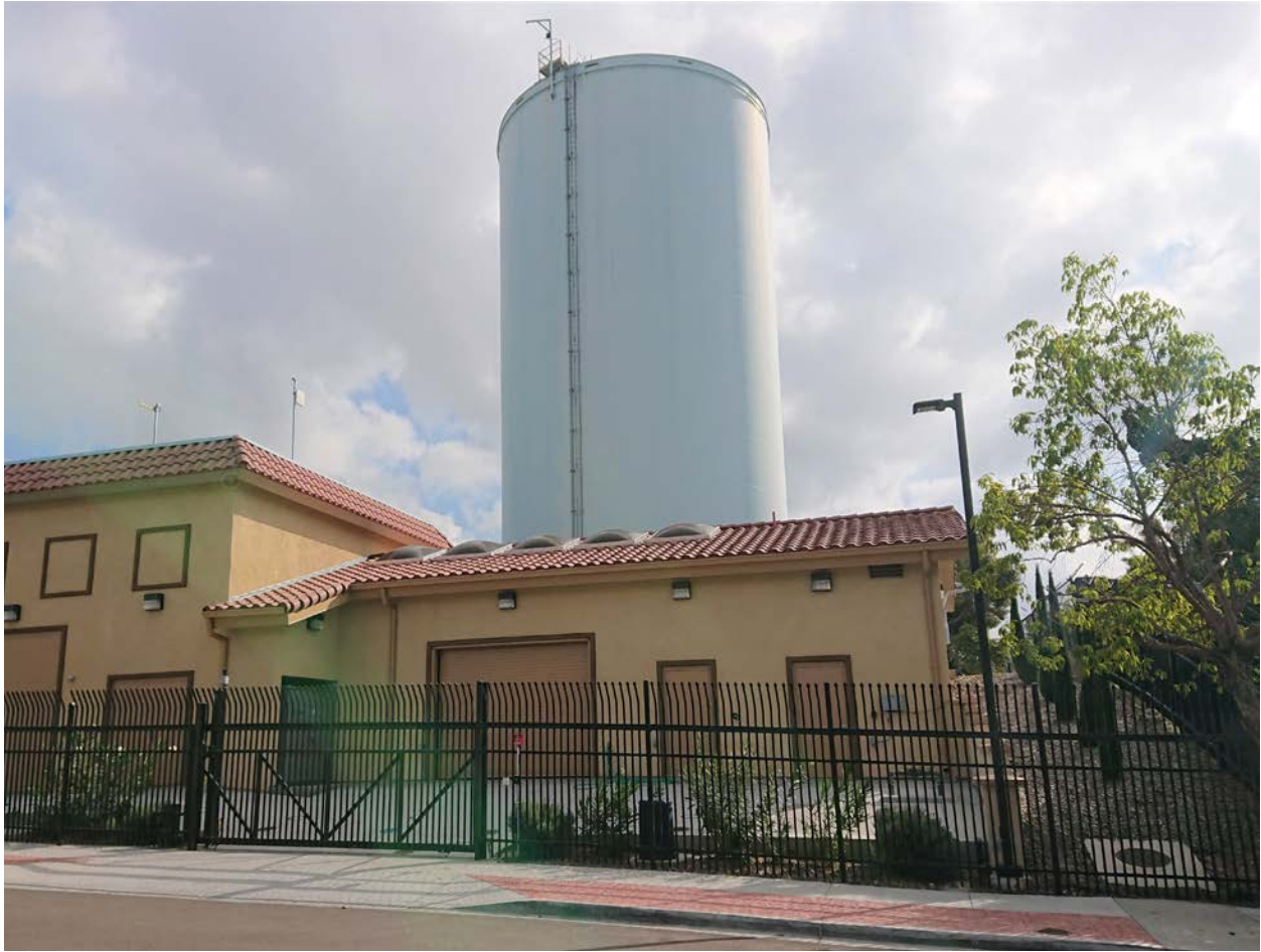
The Navajo Pump Station was constructed in 2024 to replace the College Ranch Hydro Pump Station.
