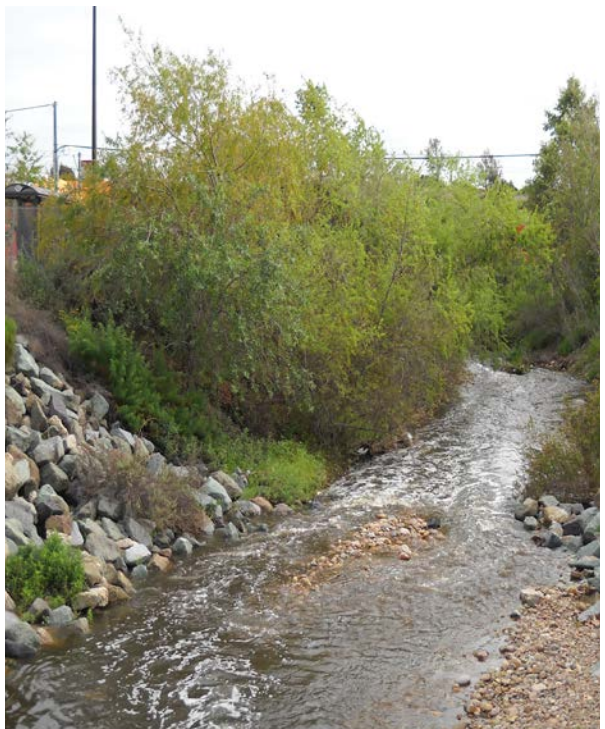
The Chollas Creek restoration in Southeastern functions as a Low Impact Development strategy.
