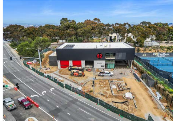
Fire Station 52 under construction near the UC San Diego campus.
