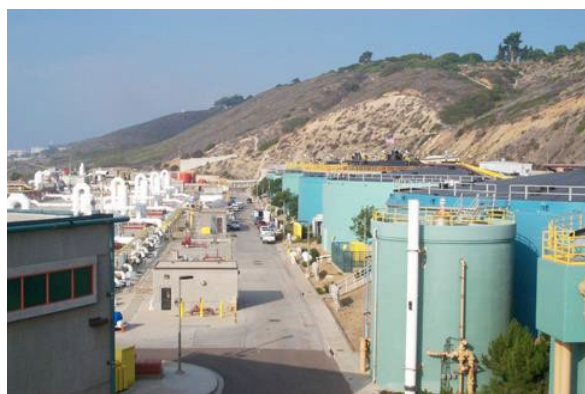
Point Loma Wastewater Treatment Plant
