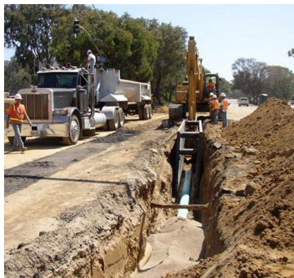
Trenching the municipal sewer.
