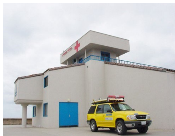
Lifeguard towers are located throughout coastal areas.
