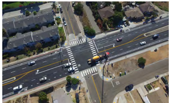
Before (above) and after (below) photos of a street redesign in the Chollas Triangle section of the Eastern Area.
