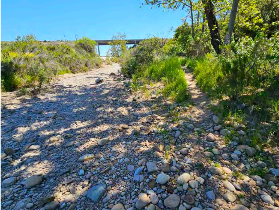
Photo 10. View to the east showing how the existing informal trail runs straight into the streambed in the bottom of Rose Canyon. Any effort to establish a formal trail here would require impacting the streambed and/or adjacent sensitive habitats (see Photos 9, 11).
