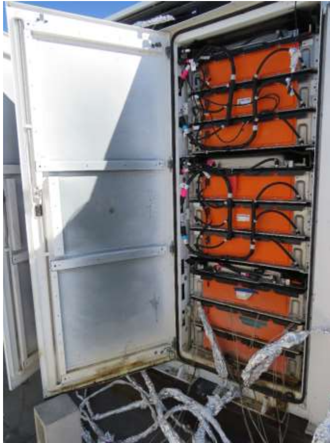
Fig 9. Internal view, post test photo
