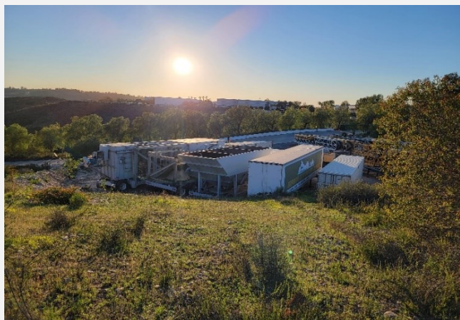
View Facing West
