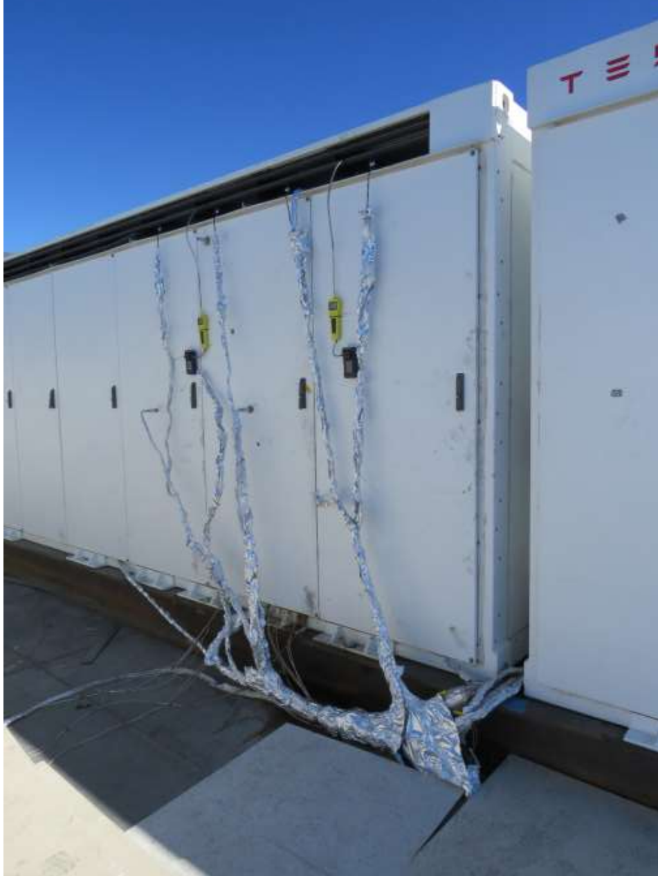
Fig 8. Post-test photo of Initiator location
