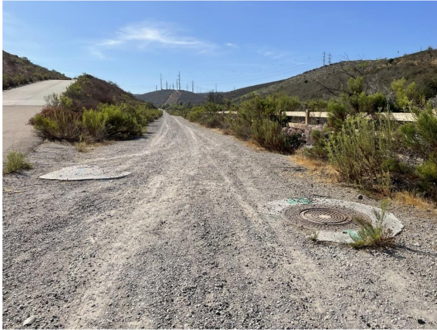
Figure 3. Overview of Green Valley Ct, looking southeast, showing buried utility access points in line with roadway
