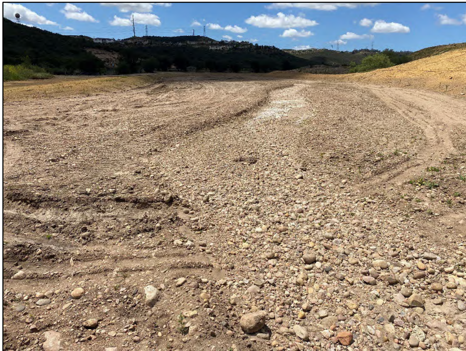
Photo Station 3-2, Facing West-Southwest (4-20-22)
