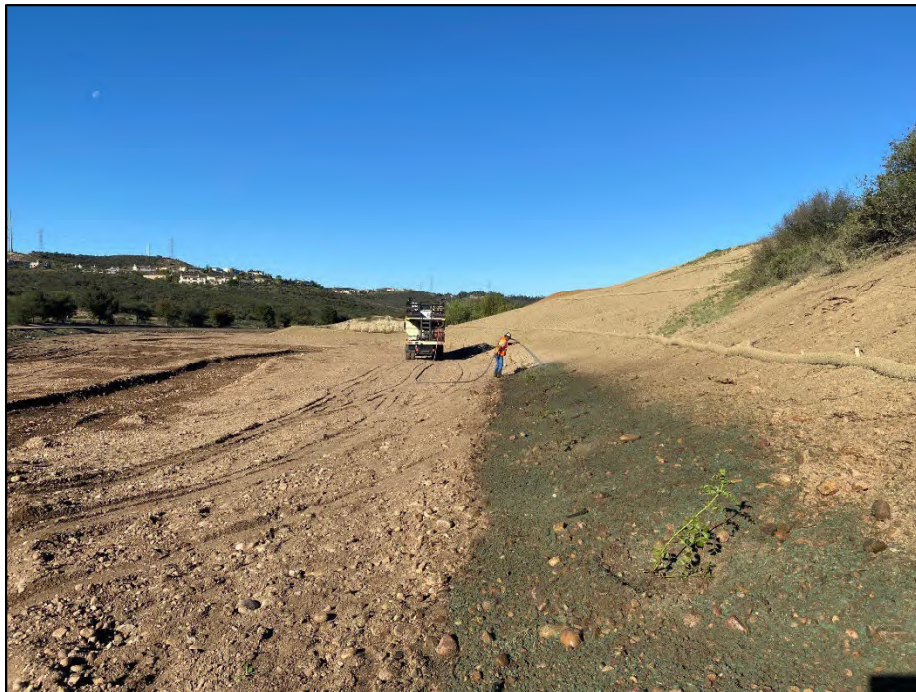
Continuation of Hydroseeding Near Container Plants (3/23/22)
