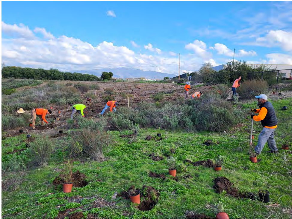
Photo 58. Contracted crew performing plant installation.
