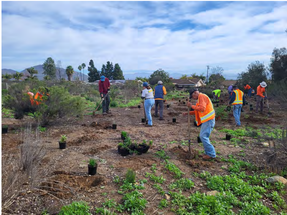
Photo 51. Contracted crew performing plant installation.
