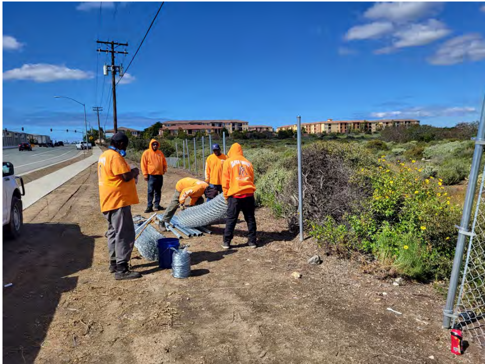
Photo 4. Contracted crew performing fence repair.
