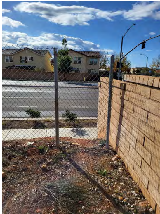
Photo 20. City staff performed fence repair.
