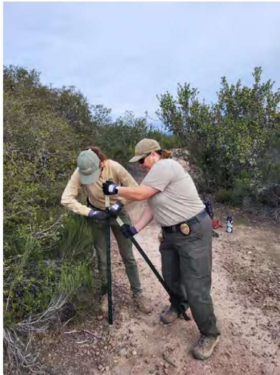
Photo 21. City staff installing fence to restrict access to vernal pools.
