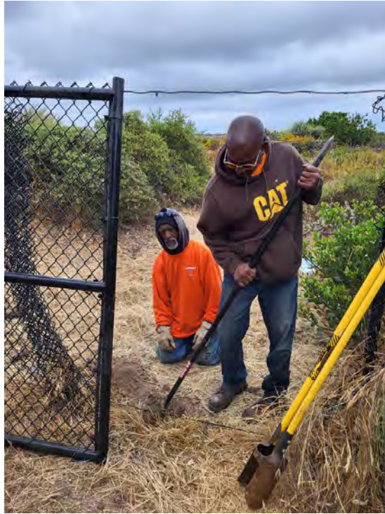
Photo 60. Contracted crew performing fence installation.
