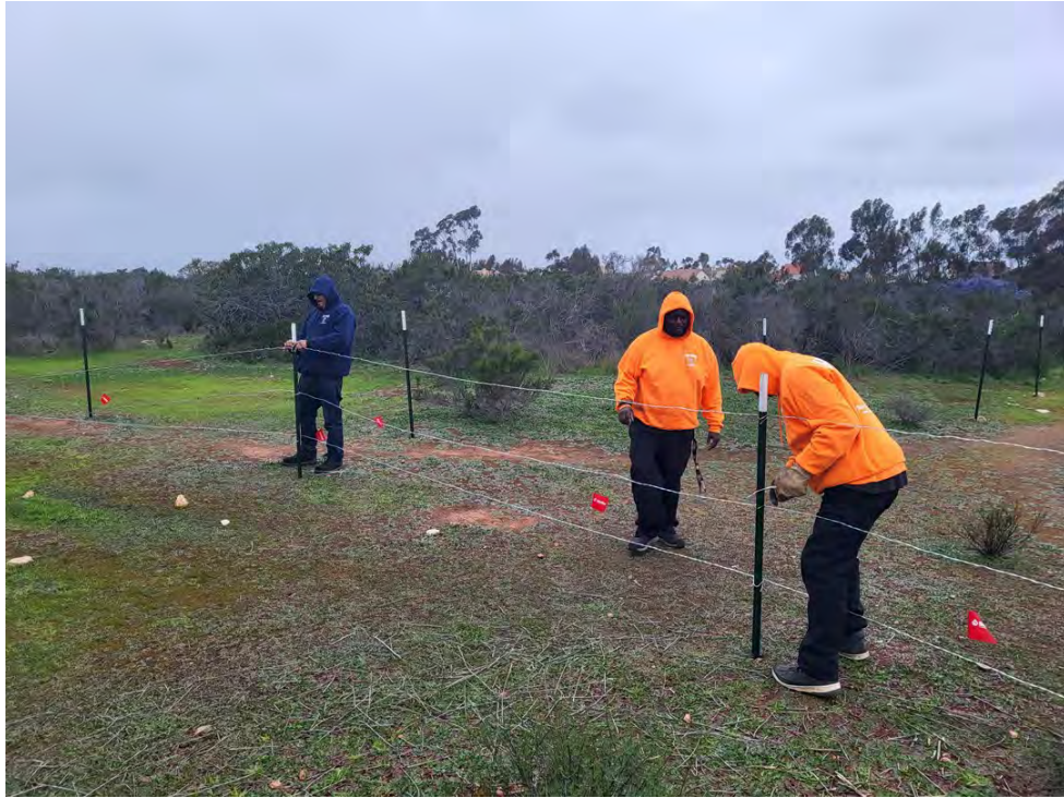
Photo 79. Contracted crew performing fence installation.
