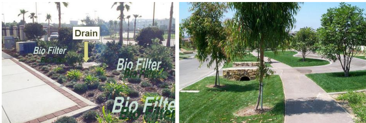
Planted areas and grass swales can serve to treat adjacent impervious areas.
