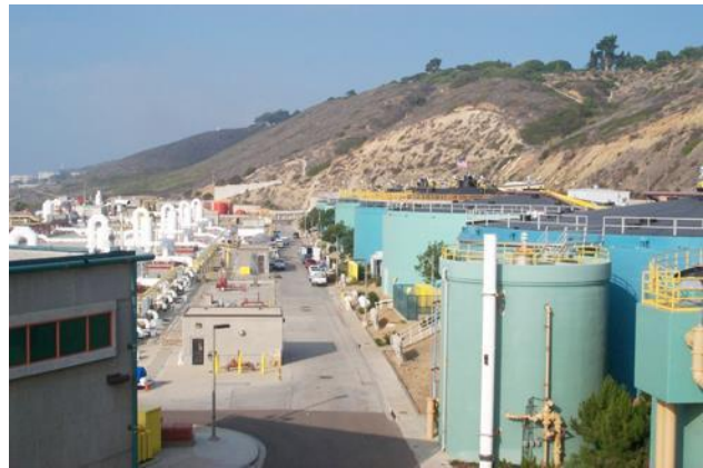
Point Loma Wastewater Treatment Plant
