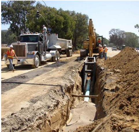
Trenching the municipal sewer system
