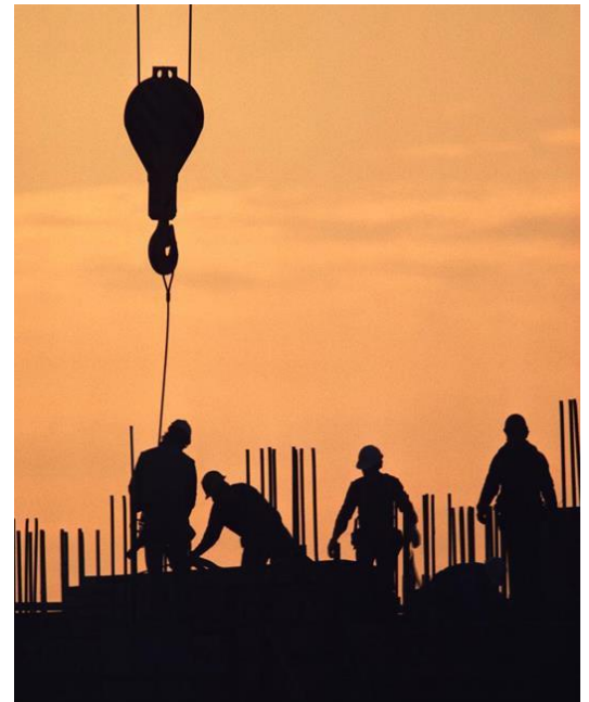
Capital improvements under construction.
