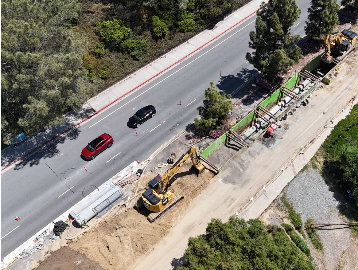
Pipeline installation on Genesee Ave.
