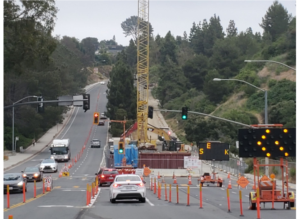
Tunneling shaft near UC High School
