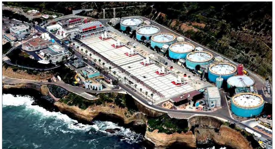
The Point Loma Wastewater Treatment Plant
