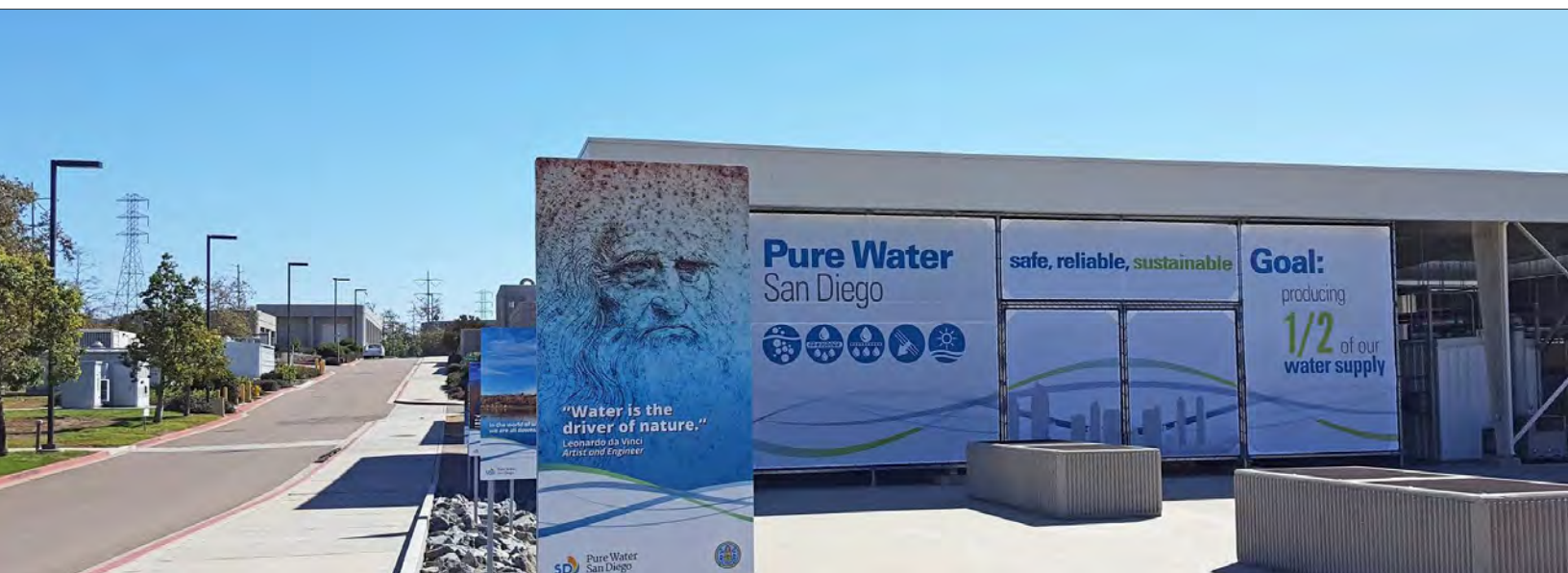
The Pure Water Demonstration Facility
