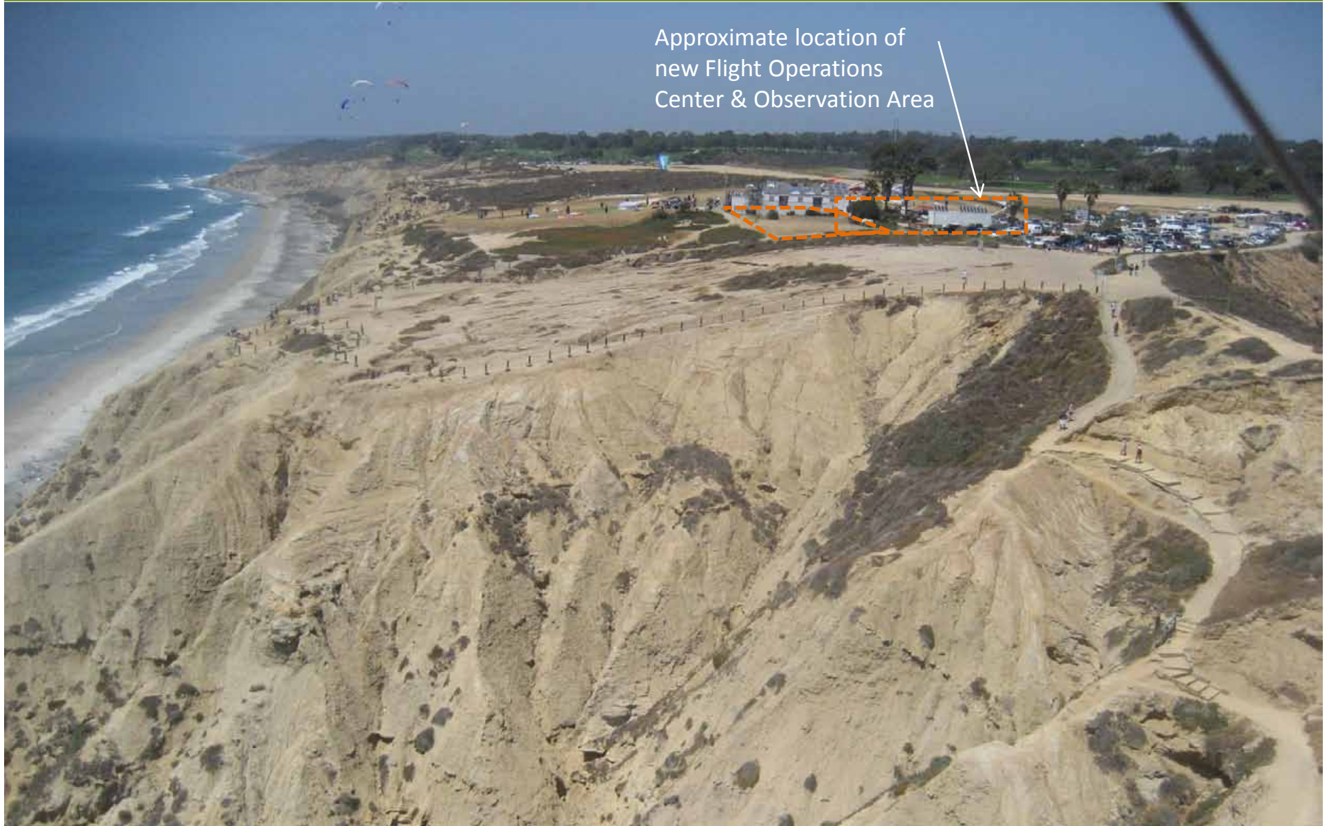
South Bluff - Existing Condition
