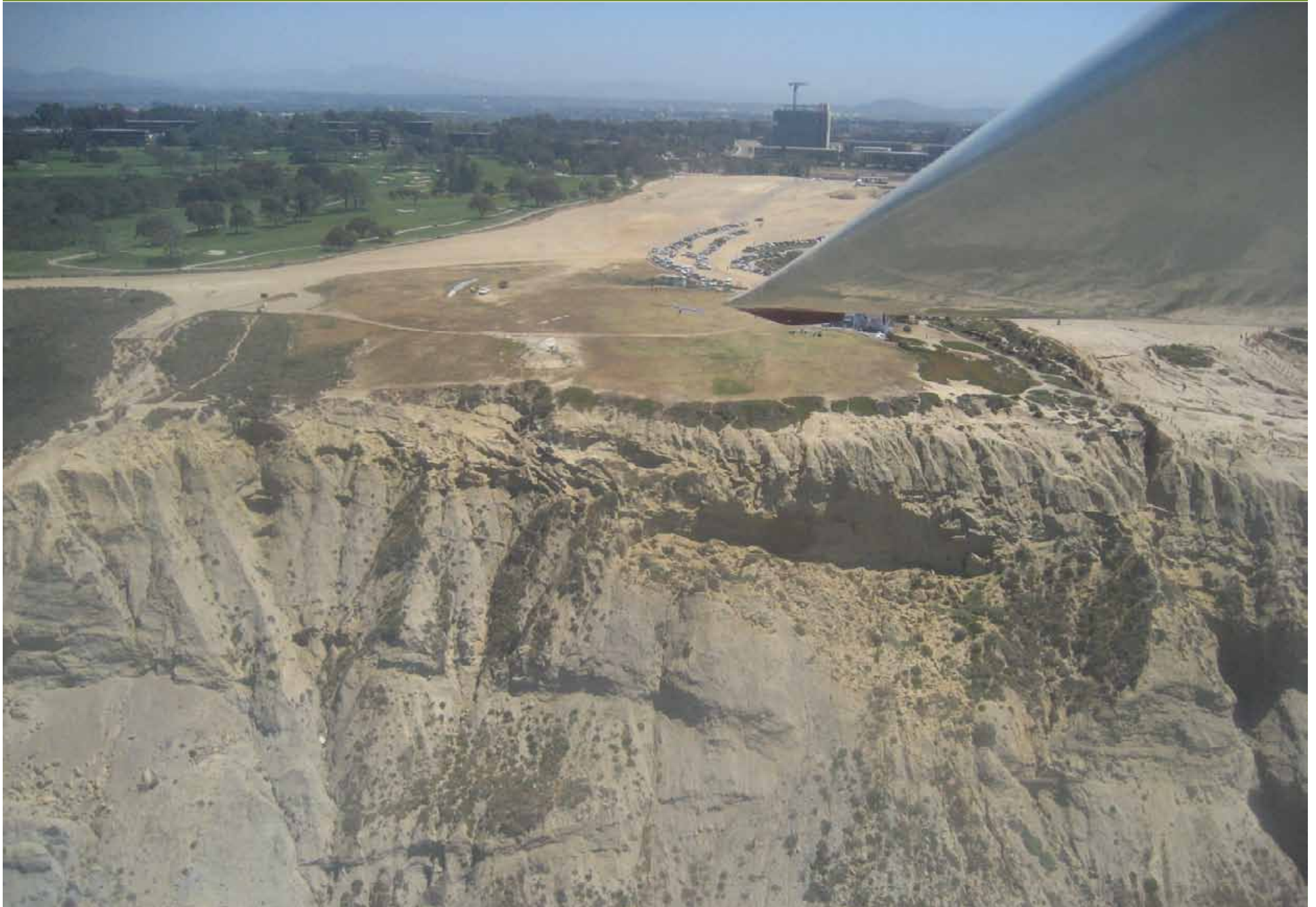
Airfield – Existing Condition
