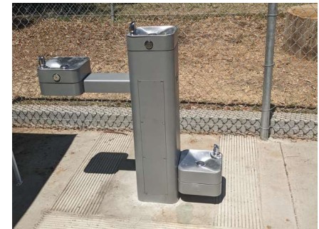
Dog drinking fountain (TBD). Contingent on funding and access to potable water line.
