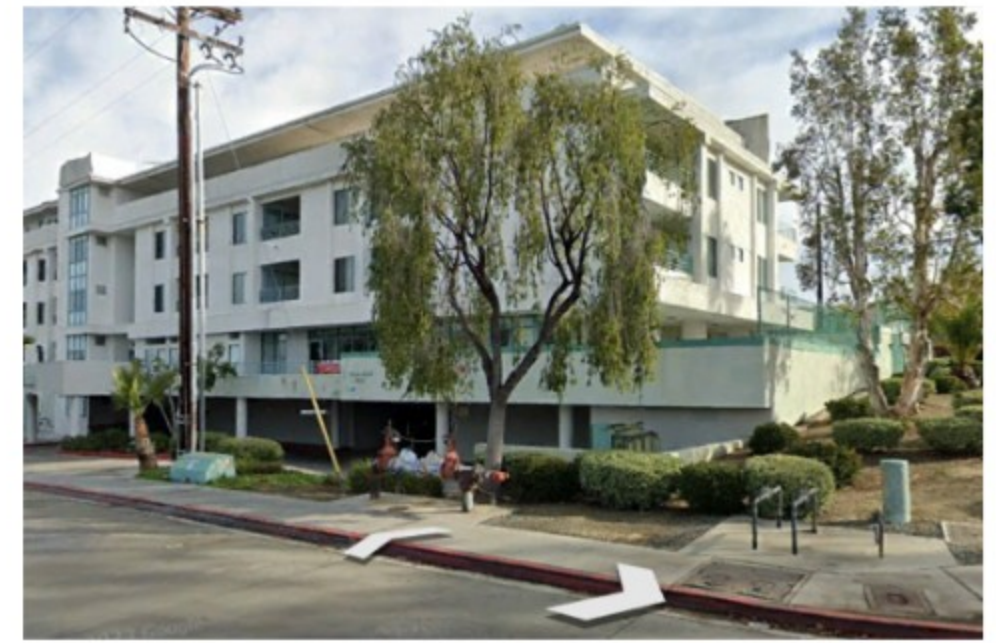
An example of a multi-family housing development within a superblock in the Colina Park neighborhood of City Heights.
