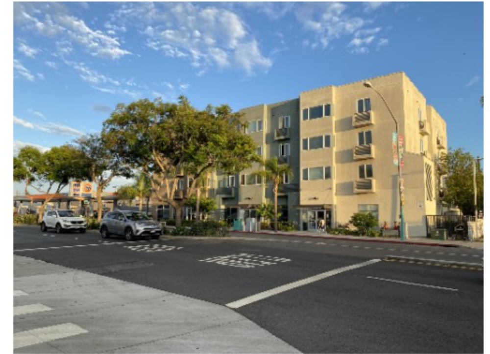
A medium density housing project near El Cajon Boulevard
