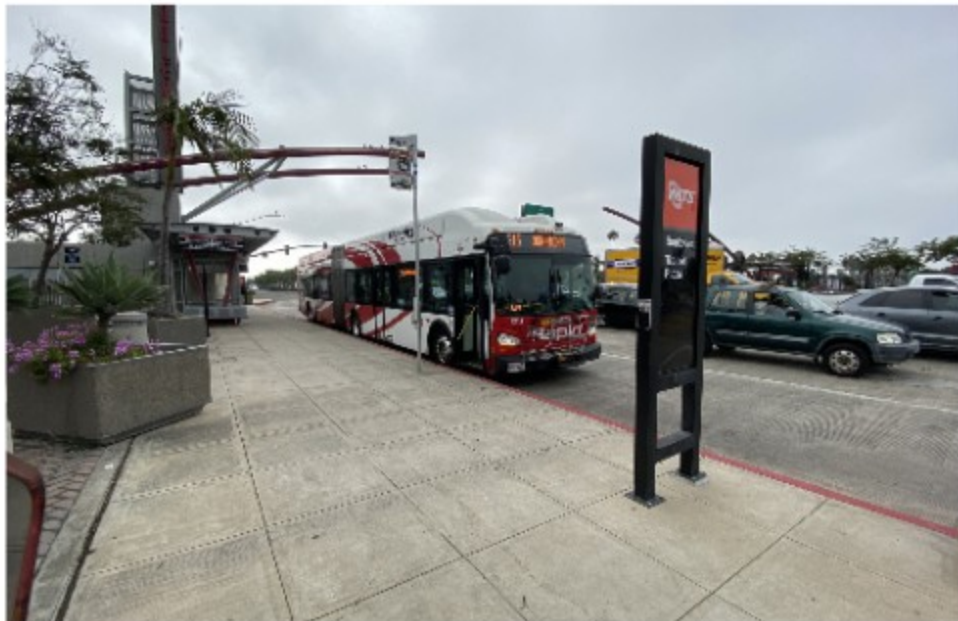
Boulevard Transit Plaza
