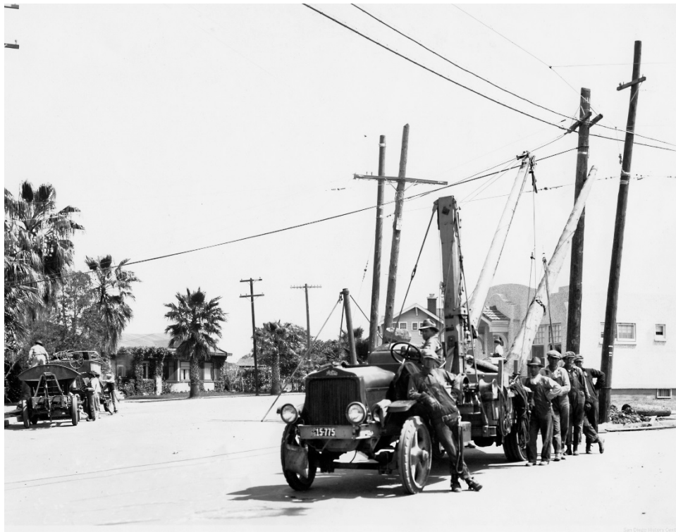
Figure 12. Electrical pole maintenance and replacement on Adams Avenue with Panorama Drive in the background, 1924 (San Diego History Center)
