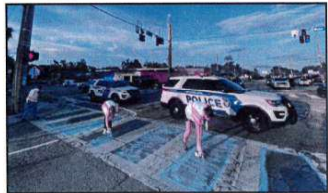
Kittelerson staff installing quick build demonstration on Corinne Drive in Orlando
