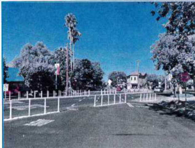
Quick Build traffic diverter with bike cut outs in Sacramento
