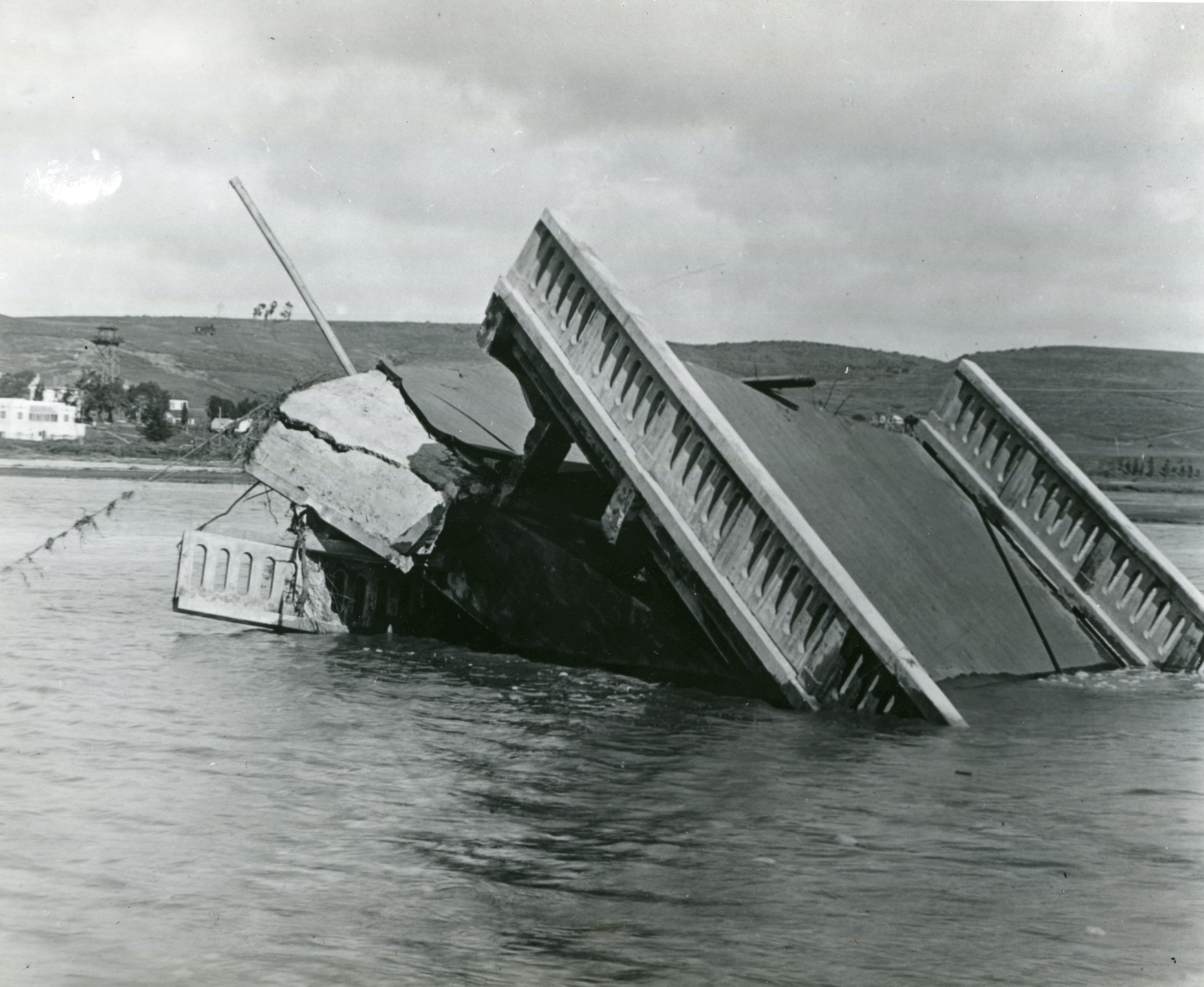
CONCRETE BRIDGE OLD TOWN July 29, 1916
