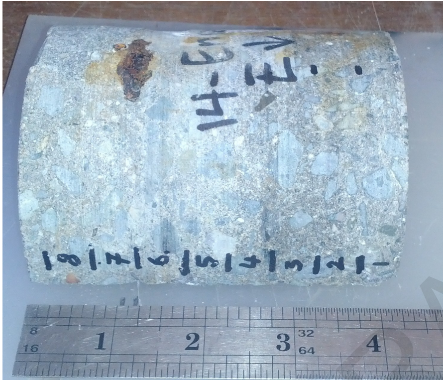
Core #14: Half core A (Pile Splash, Encasement) with embedded steel cable visible between sections 6 and 7. The 0.5” sections were cut on a tile saw with a 1/16” blade.
