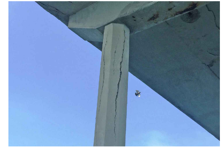
PILE DAMAGE
