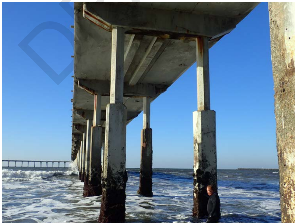
Figure 4 - Concrete Encasements at Bent 12
