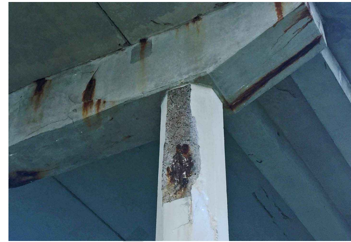
PILE DAMAGE
