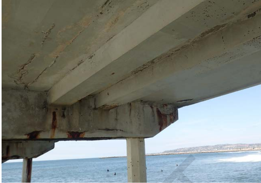
Figure 21 - Cast-in-place Beam Repair
