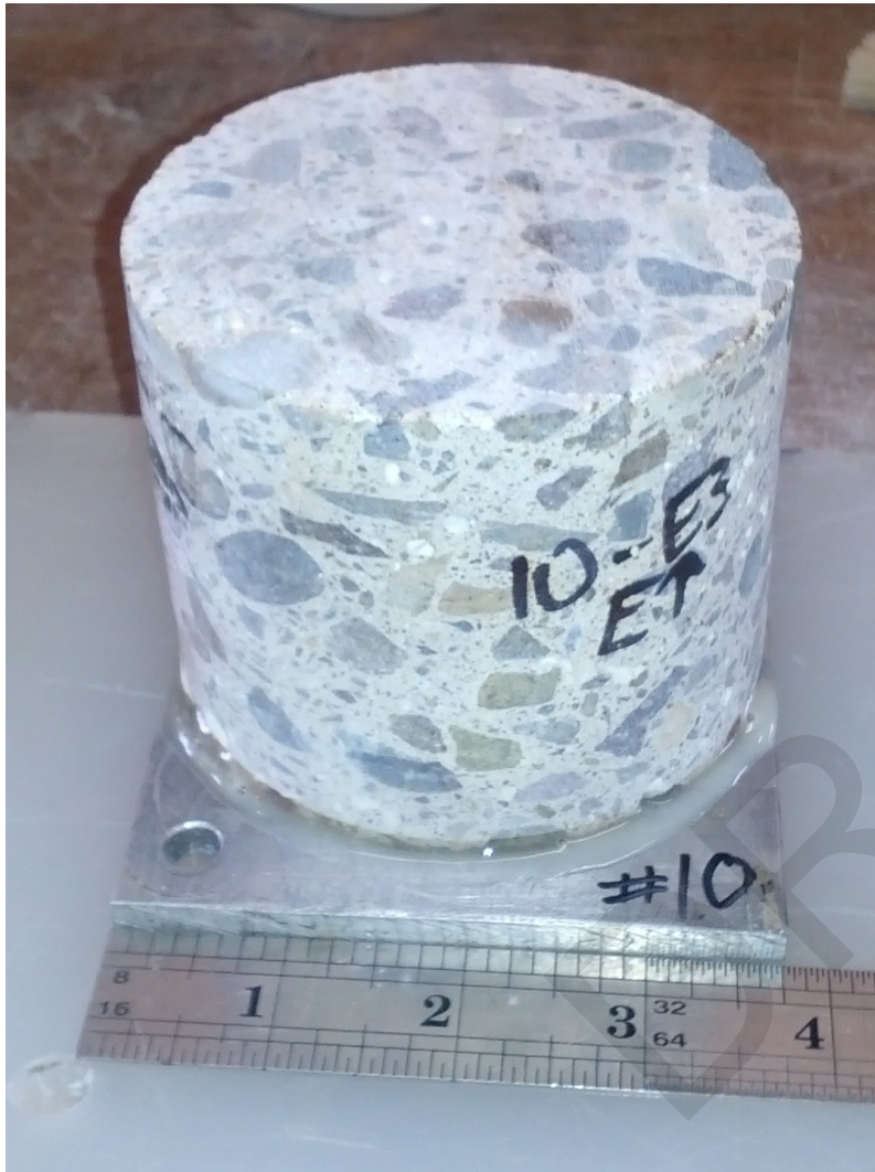
Core #10: Section for chloride analysis was cut at 2 1/2" from the exposure surface. No reinforcement was observed.
