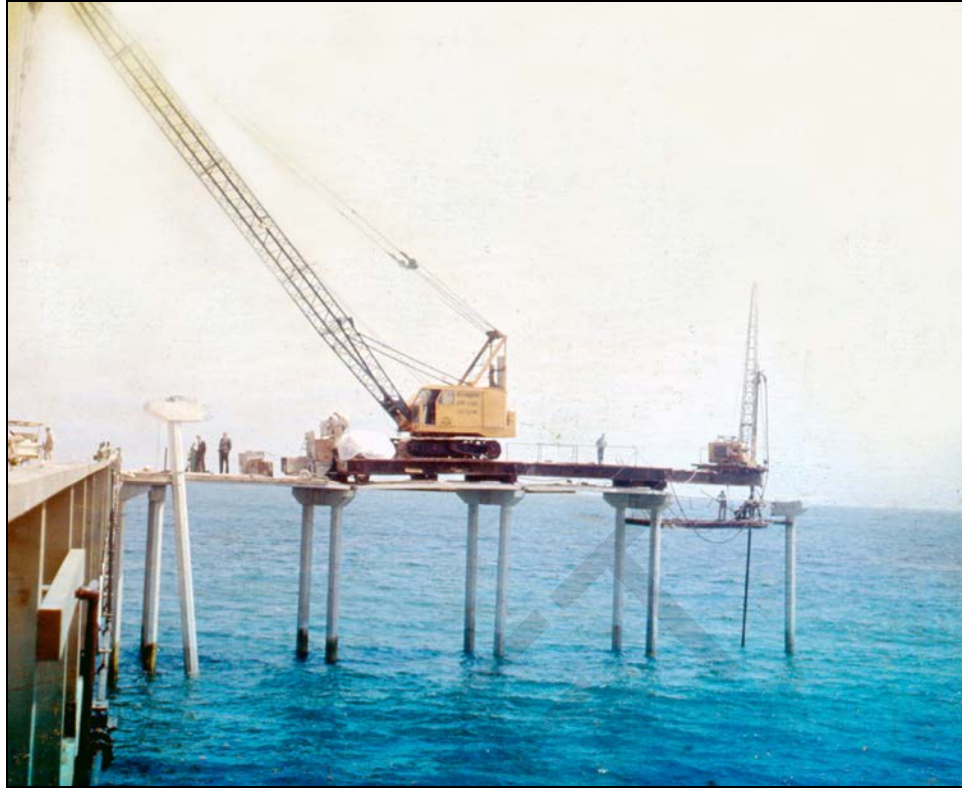
Figure 1 - North leg of the pier under construction
