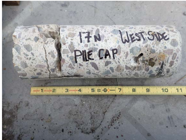
Figure 7 - Example concrete core from Pile Cap 17N
