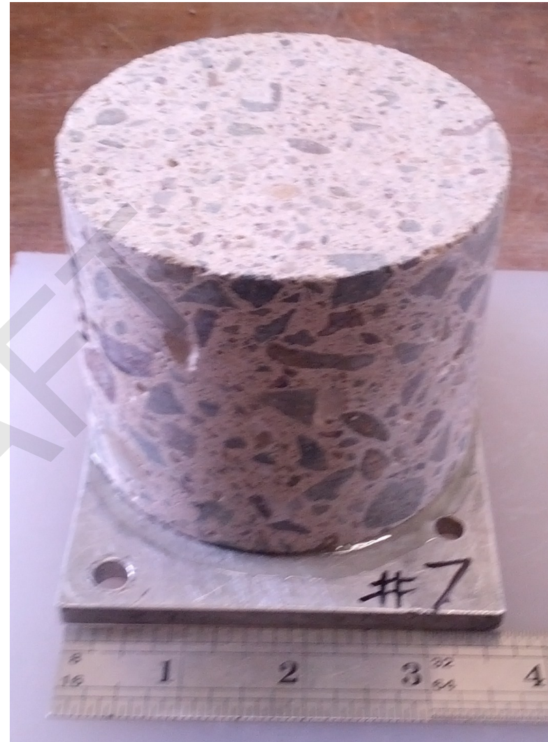
Core #7: Section for chloride analysis was cut at 2 1/2" from the exposure surface. No reinforcement was observed.
