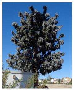
Figure 21: A mono-pine. Note how difficult it is to see the antennas.
