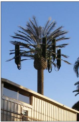
Figure 32: Faux palms do not provide the level of concealment required by the Wireless Ordinance - they are monopoles with fronds!
