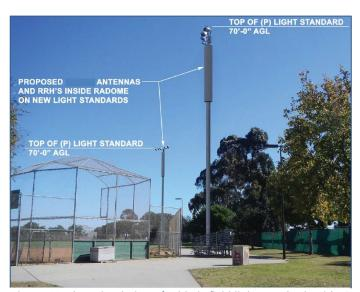
Figure 11: Photosimulation of athletic field light standards with antenna shrouds.
