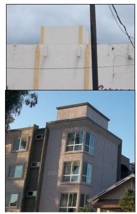
Figure 28: Two rooftop boxes that replicate existing building elements well.
