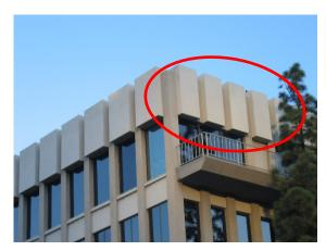
Figure 1: A well-concealed WCF. Antennas are architecturally integrated into the building.
