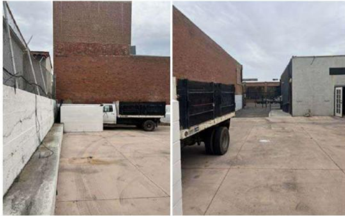
⑥ (E) OUTDOOR PATIO - NORTHEAST SIDE
