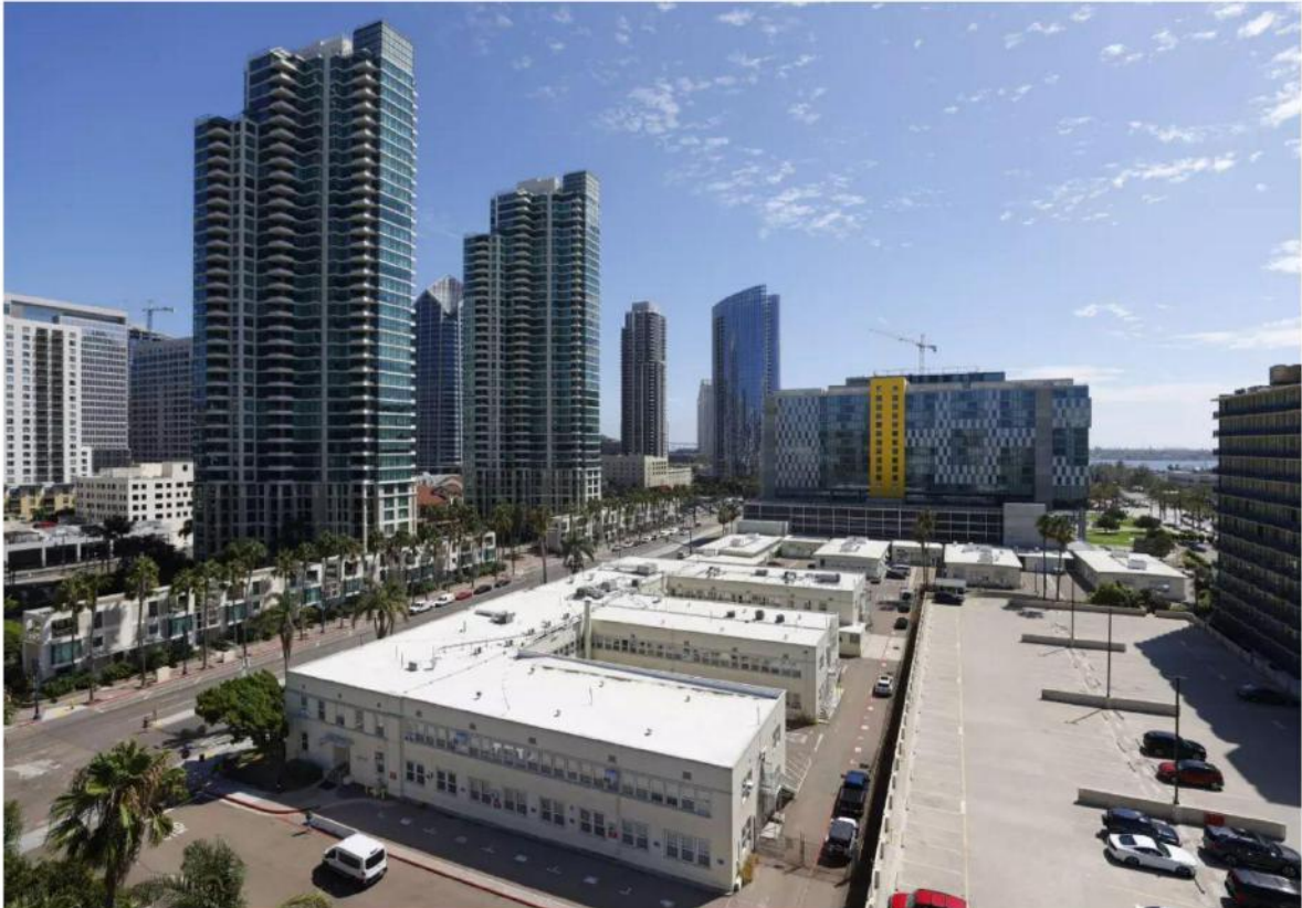
Sandwiched between the Wyndham San Diego Bayfront hotel and the Lane Field hotels, the low-rise buildings at 1220 Pacific Highway are the property of the United States Navy. The Navy has agreed to terminate its 100-year lease with the Port of San Diego for the 3.4-acre property. (K.C. Alfred/The San Diego Union-Tribune)
