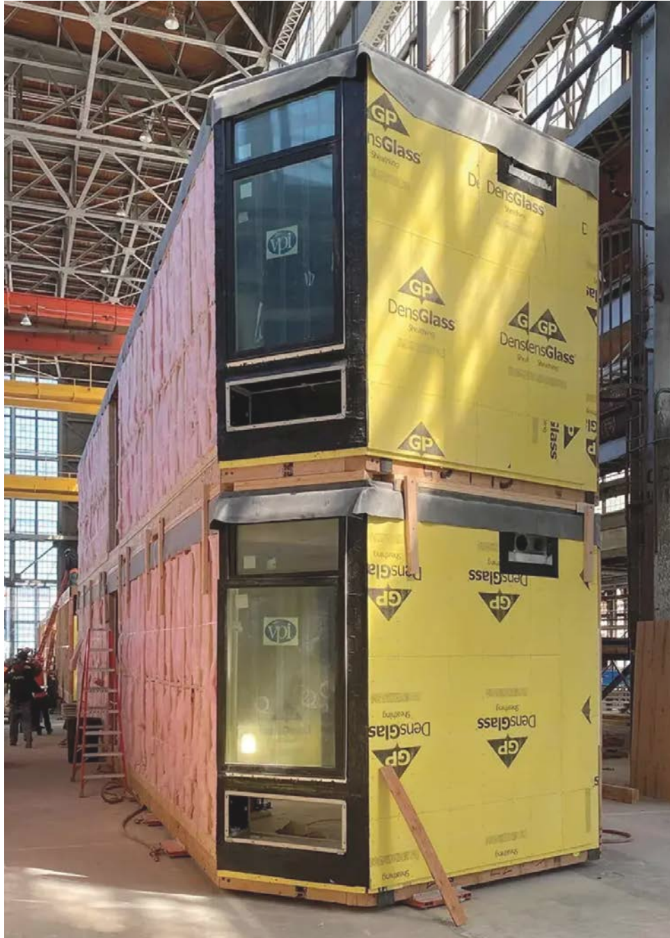
1. Modules are pre-fabricated in a factory to reduce on-site construction time
