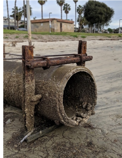
Figure 14. A coastal storm water outfall in San Diego.
